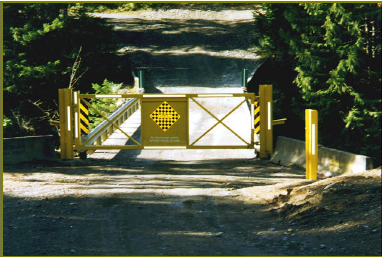
Plate 7: Access Gate at Burnt Bridge
