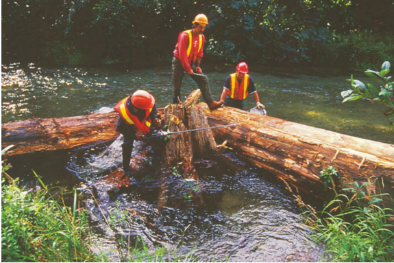
Figure 2. Post-construction view of Snootli Creek site.
