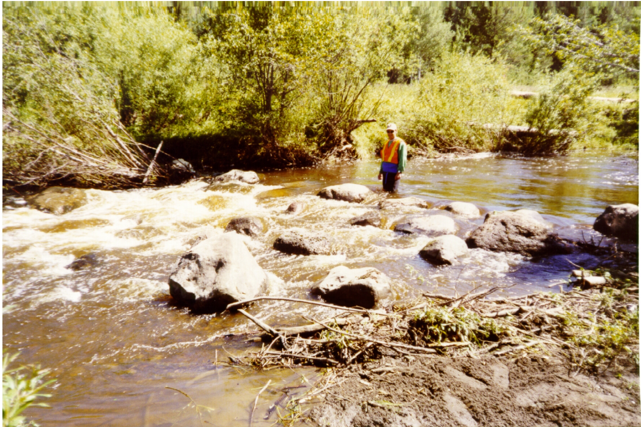
Figure 1: Rock riffle construction on the Clisbako River, Cariboo Region.
