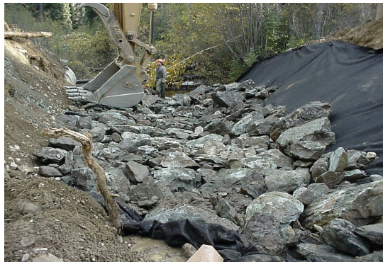
Figure 4 Rip-rap placed on top of geotextile
