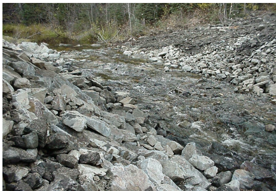
Figure 5 Prepared stream bed after culvert removed
