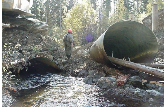
Figure 2 Diversion into one culvert
