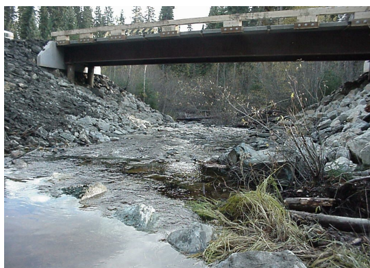
Figure 6 Bridge installed, channel completed
