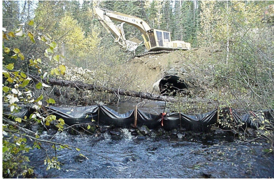
Figure 1 Silt fence downstream
