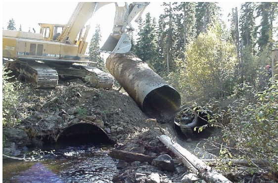
Figure 3 Lifting first culvert
