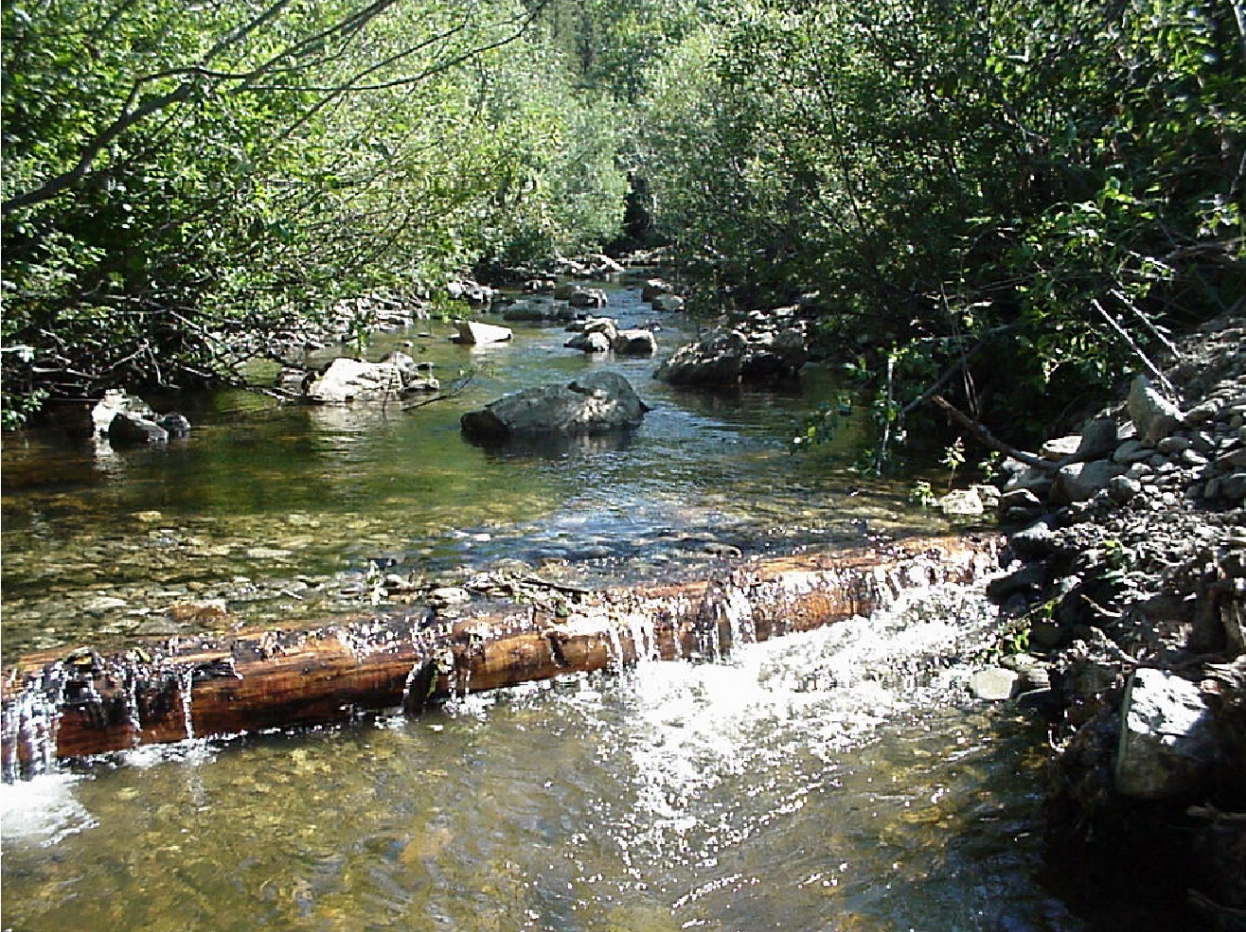
Figure 2: Fontaine Creek Site E: Upstream view of LWD scour log and boulder clusters placed to restore pool habitat.
