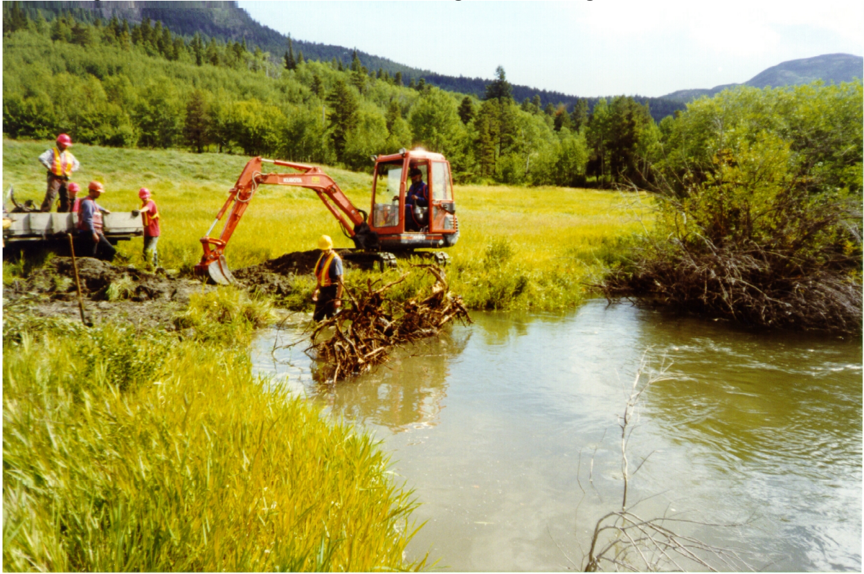
Figure 1: Installation of LWD revetement during late summer high flow, Homathko River.
