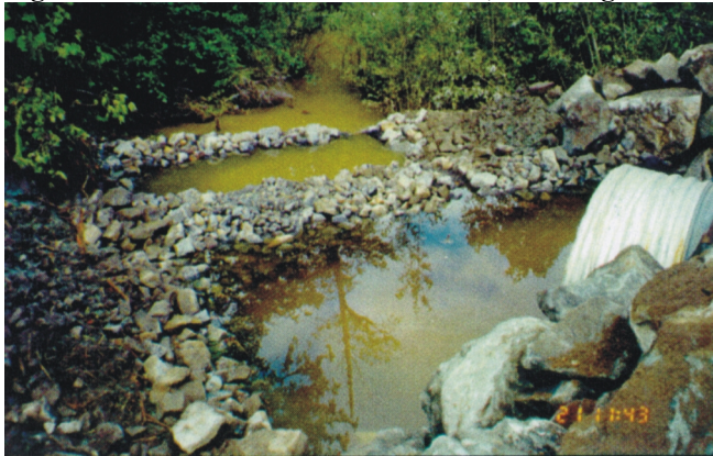
Figure 1: Site MM 07 – view of culvert, retaining weirs and the resulting pools.
