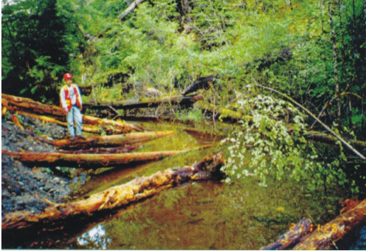
Figure 2: Site MM07 – view of excavated pool with LWD positioned at approximately 40° angle.
