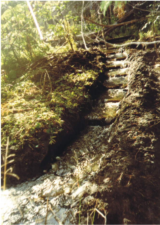
Figure 2: A series of fry accessible ladders were constructed around old, non-active, beaver impoundments, to access groundwater rearing habitat in the glacial fed Talchako river system.
