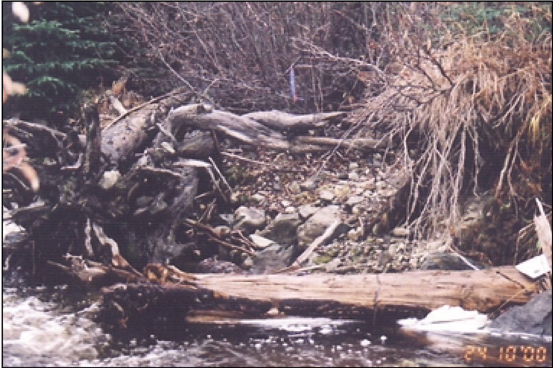
Photo 3: Rebman Creek Site 2: left bank LWD structure, Reach 2 at ~1,505 m.
