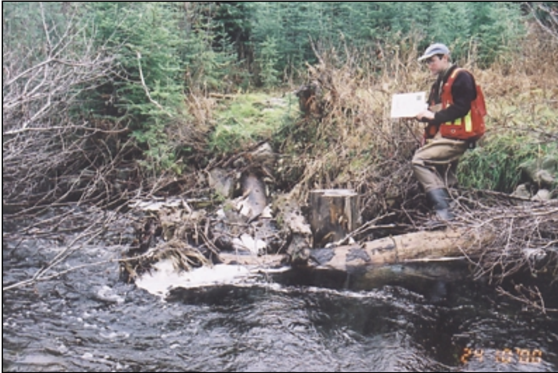
Photo 23: Rebman Creek Site 12: left bank LWD structure, Reach 2 at ~2,096 m.
