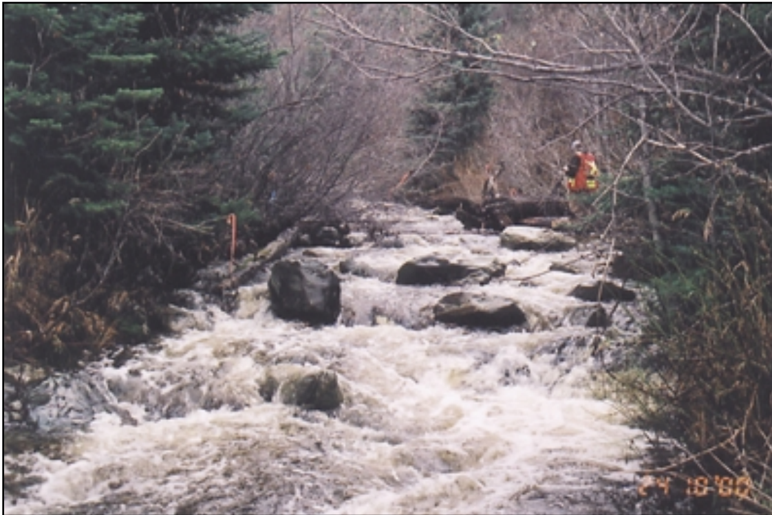
Photo 14: Rebman Creek Site 7: view upstream toward constructed riffle, Reach 2 at ~1,675 m.
