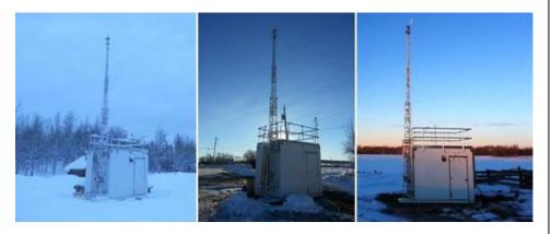
Three portable, continuous air quality monitoring stations operated at Tomslake, Doig River and Farmington in the Peace region in 2015. These stations were loaded onto a truck and transported in 2015 and 2016 to new sampling locations.
