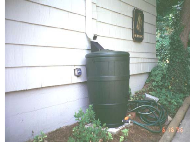
Figure 7-28a Rainwater Re-use using Rain Barrels
