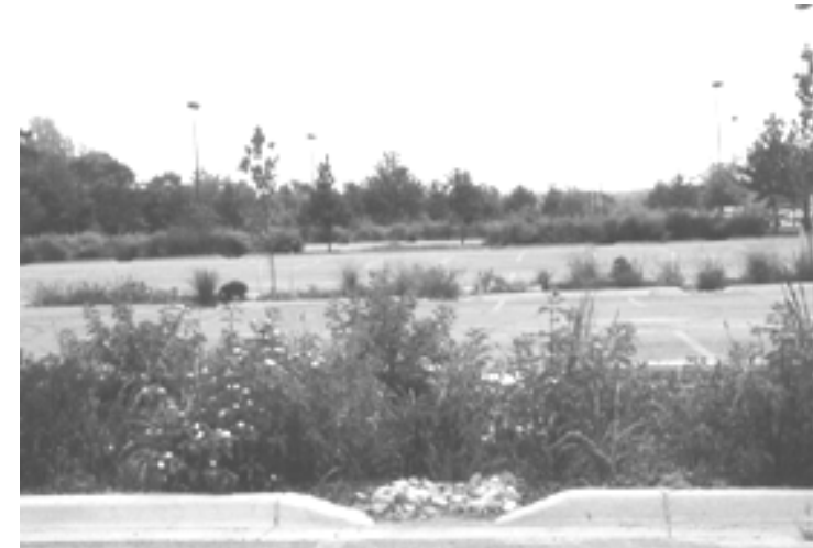
Figure 7-8b Bioretention for a Parking Lot
