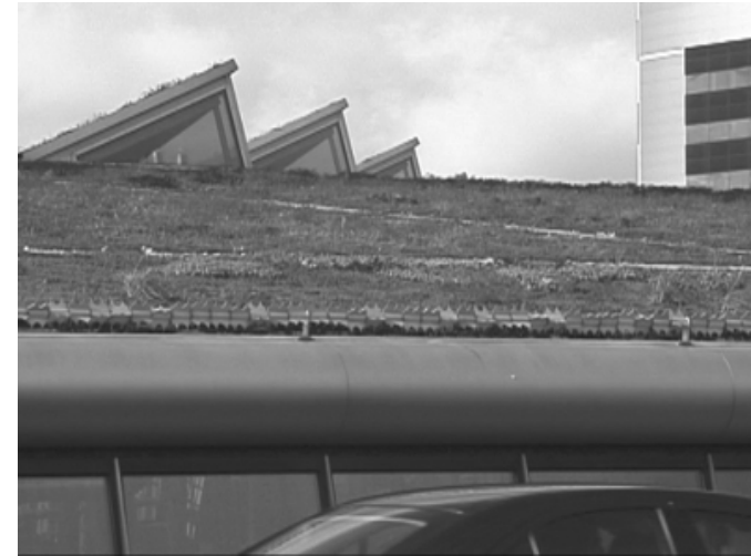
Figure 7-23 Lightweight Extensive Green Roof
