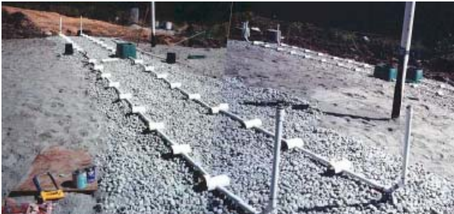
Figure 2: Installation of a ground disposal field.
