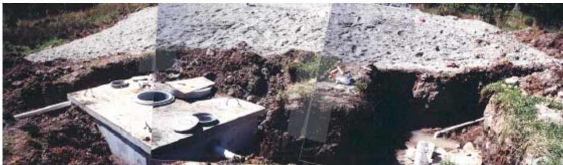
Figure 5: Installation of a septic tank.
