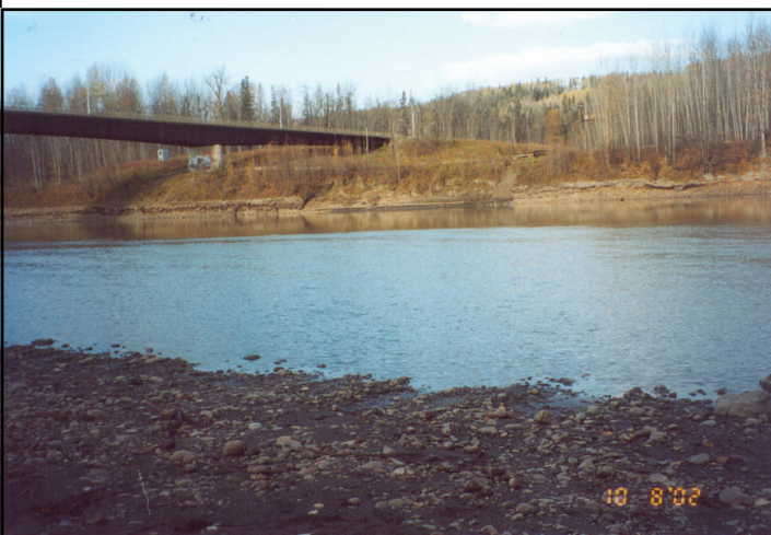
Plate 1. A view of the Muskwa River downstream of the Alaska Highway bridge. The pump house is located directly across the river from this view.
