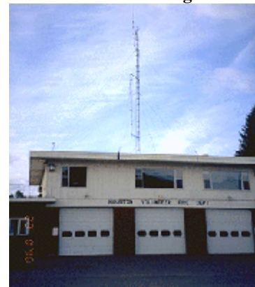
Figure 5. Firehall Monitoring Site
