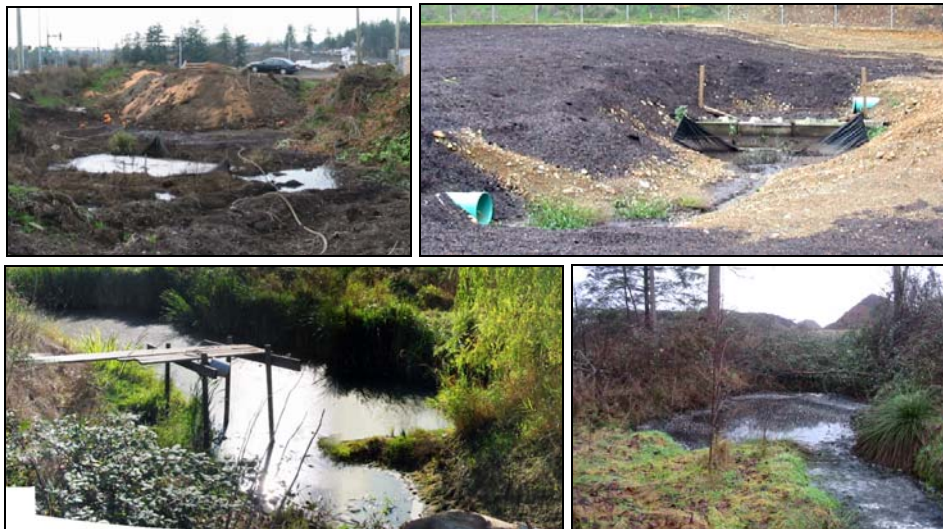
Figure 5 Leachate collection ponds at various sites. EPO's inspection assessments were that ponds are generally poorly constructed and/or maintained as there is no documentation that the underlying soil is impermeable and/or they appear to overflow in wet weather.
