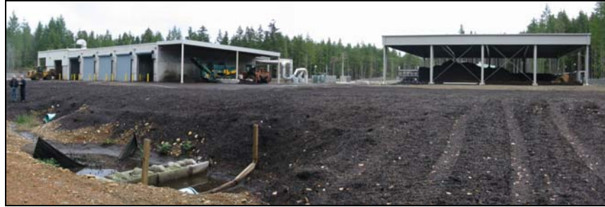
Figure 4 The Site H in-vessel composting facility. To the left is the compost building housing the mixing, composting bins and screening facilities. To the right is the curing building. A leachate collection pond is shown in the lower left of the photo.
