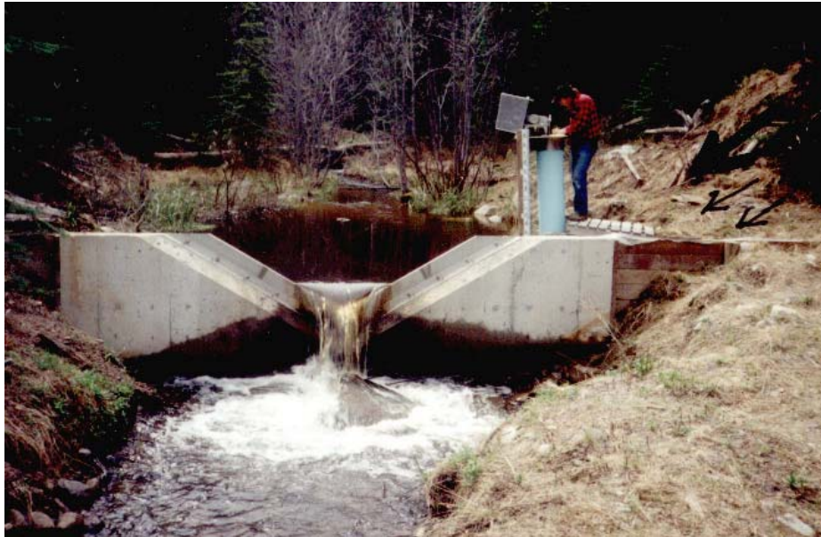
Figure 65: Stilling well installed in the weir pond.
