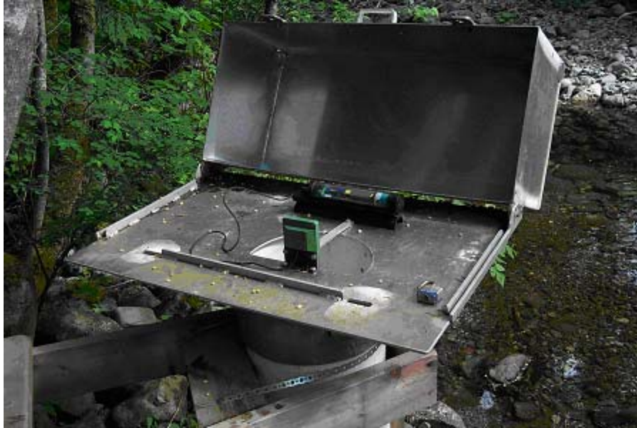
Figure 30: Thalimedes (Shaft Encoder) installed in 12" ABS. This site originally set up with Stevens A71 Chart Recorder. Thalimedes used to retrofit existing well and shelter.
