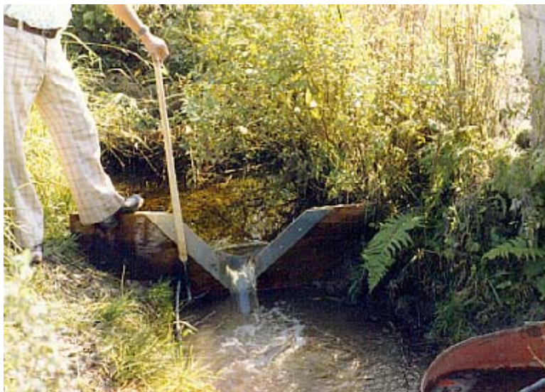
Figure 74: V-notch weir plate, portable installation.
