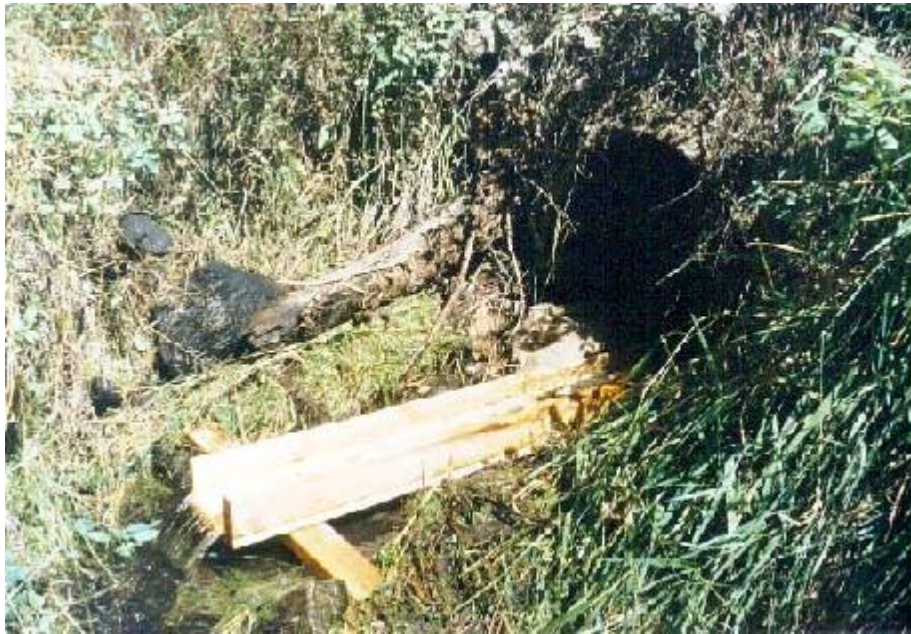
Figure 69: Culvert with low outlet and flow led into flume for volumetric measurement.
