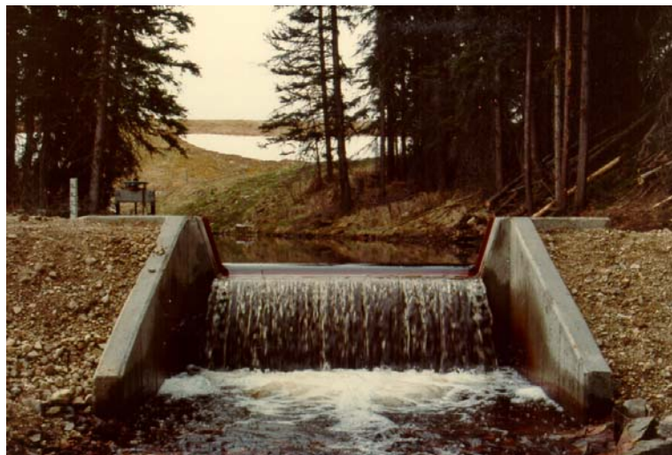
Figure 4: A Stable artificial control (weir).
