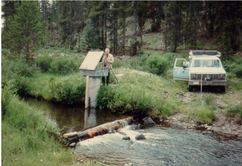
Figure 5: A Stable artificial control (log sill).
