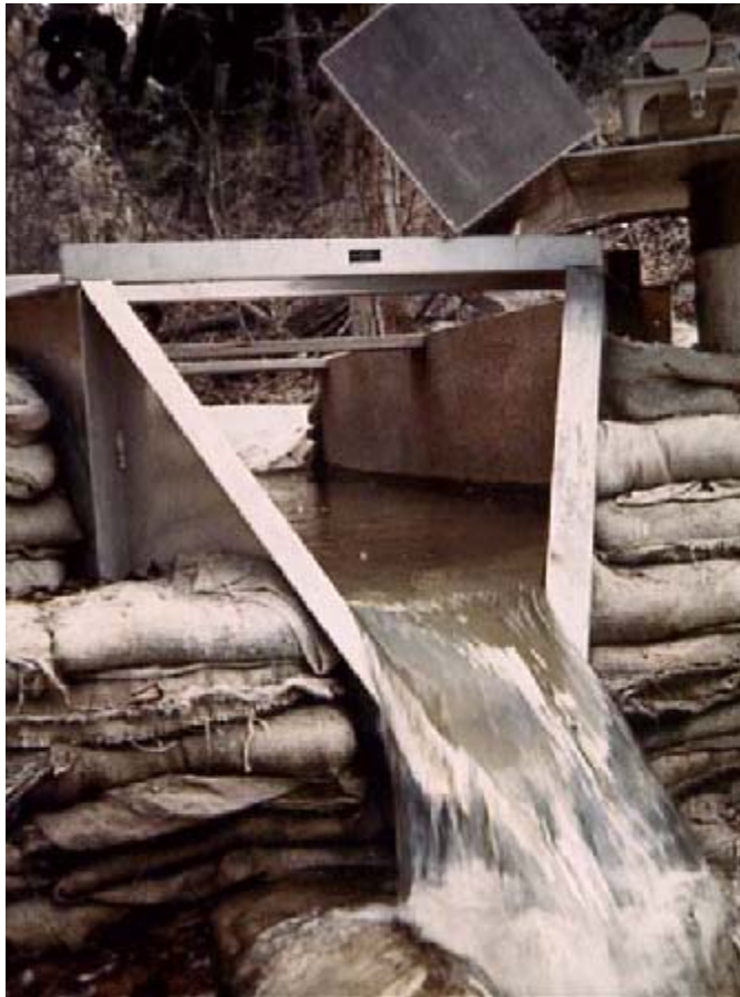
Figure 63: 2.5 foot H Flume set in concrete filled sacks. Cuisson Creek above Gibraltar Mine.
