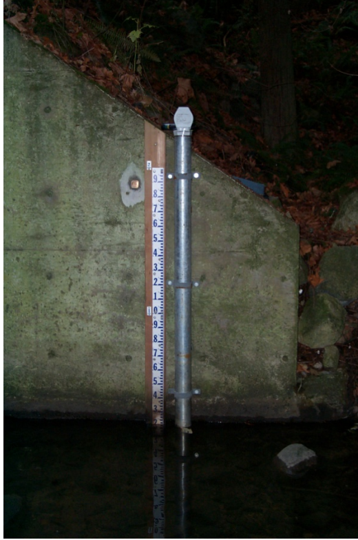
Figure 7: Gauge plate and in-stream recorder (data logger) installation. (Note the brass tablet 'bench mark' located near the top of the gauge)
