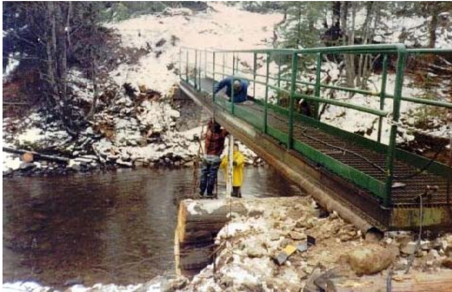
Figure 6: Trout Creek metering bridge.
