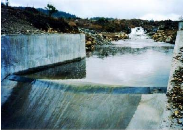
Figure 71: Pool formed by a modified Crump Weir, where both a digital and an analogue recorder are installed.
