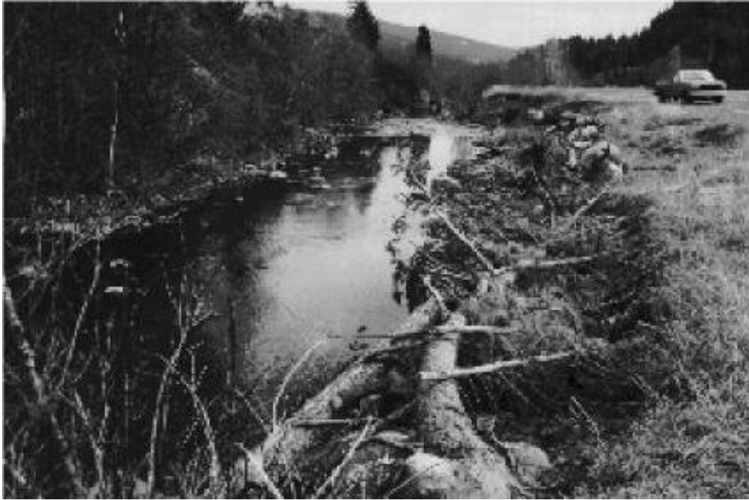
Figure 1. Typical river spur structure using large wood pieces, thinned trees, root wads and boulders; supplemented by planting willow stakes.
