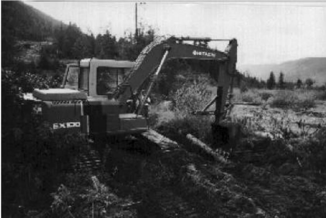
Figure 3. Excavator used to tighten and place deadman logs into T-trenches.
