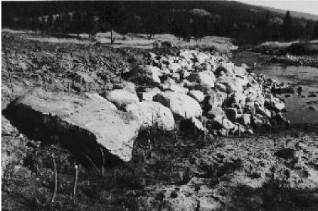
Figure 4. Channel manipulation using graded rip-rap and supplemented with planting willow stakes.
