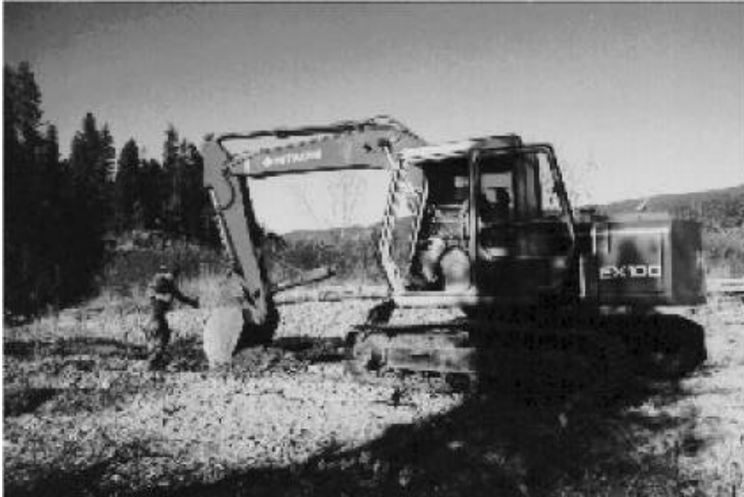
Figure 5. Bar planting using excavator 3 to 4 willow stakes were planted per bucket, up to 1 m deep.
