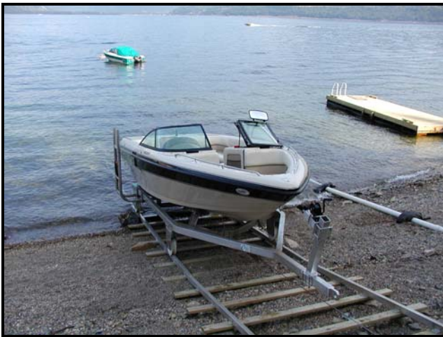
Figure 1. The system depicted requires no foreshore preparation other than minor hand relocation of foreshore substrates to level and stabilise the track. While not suitable for use on vegetated foreshore areas, due to the potential for harmful alteration of these important fish habitats, it is the preferred launch system for rock, gravel or sand foreshore areas. Each section may be lifted by two people and bolted to/unfastened from adjoining sections as water levels recede in the summer or rise in the spring, also providing for seasonal removal while not in use.
