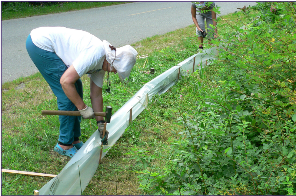
Creating fencing to divert amphibians into tunnels
