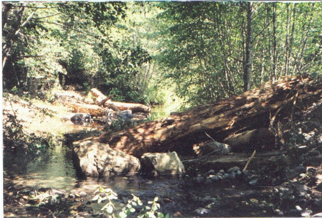
Photo 4. Looking downstream at LWD structure located at 0+101 m in Tributary G02.
