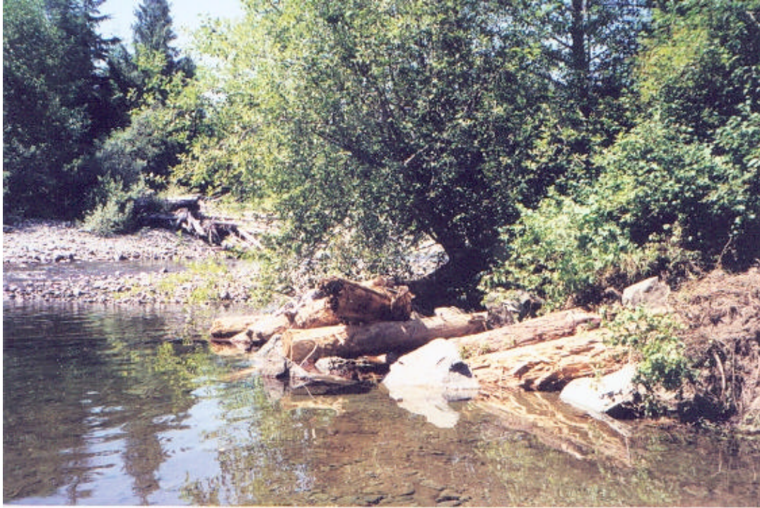
Photo 1. Looking downstream at LWD structure located at 0+000 m in Tributary G02.
