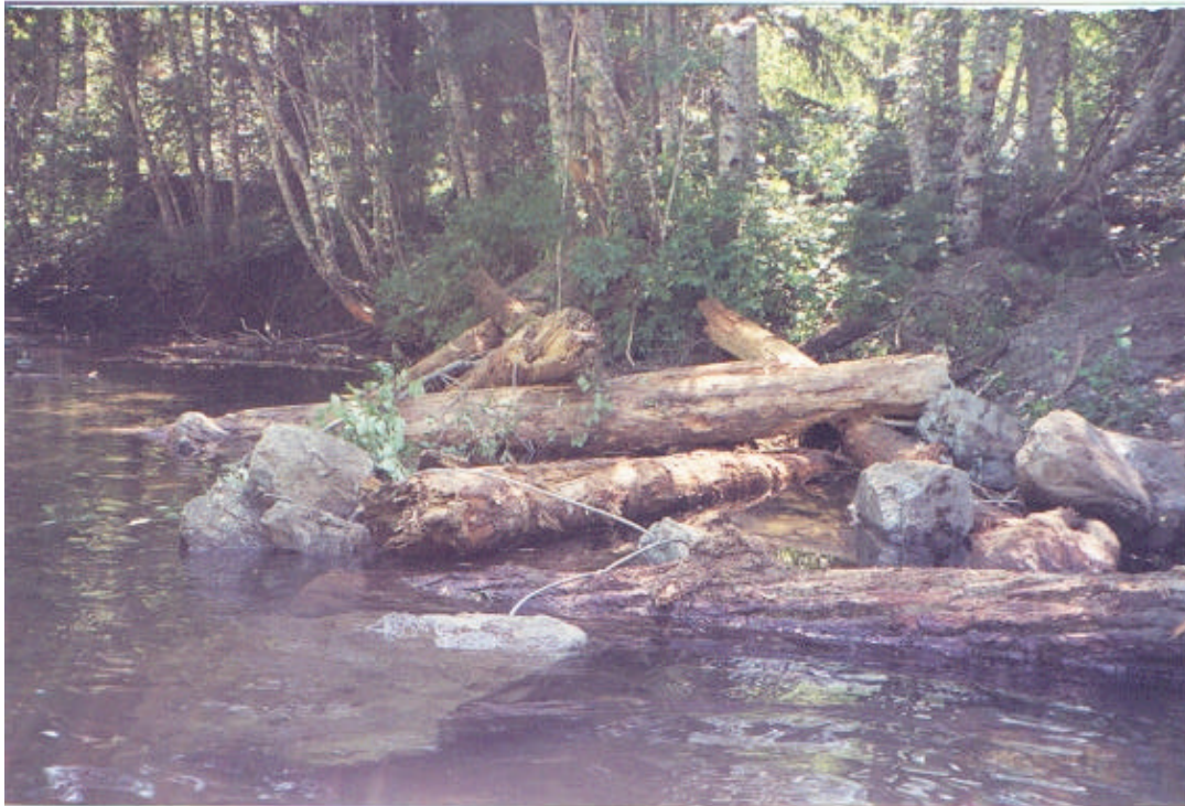
Photo 2. Looking downstream at LWD structure located at 0+038 m in Tributary G02.
