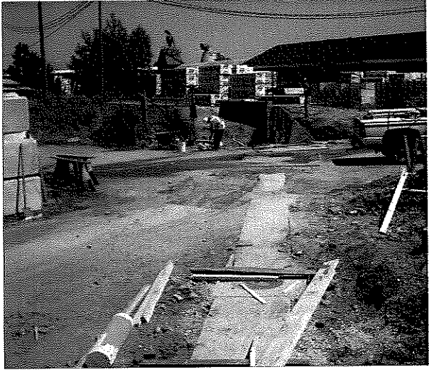
Finished buried seepage cut-off wall
