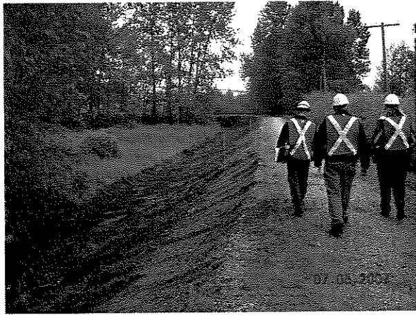
Stripping on river side of existing dyke
