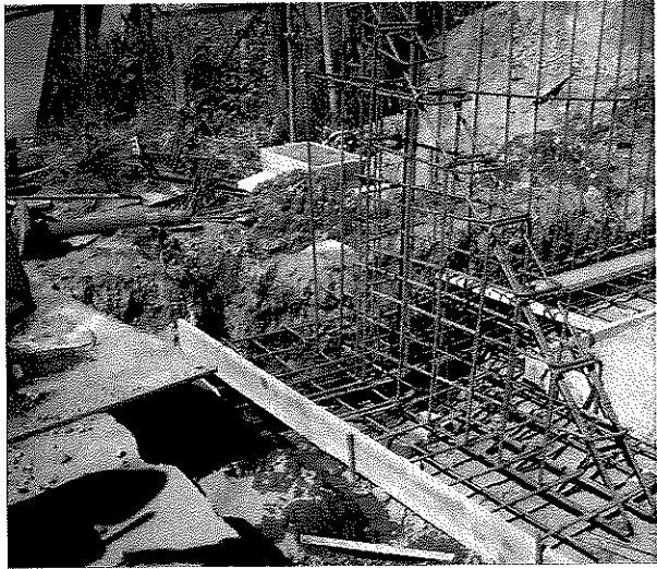
Reinforcement for abutment wing wall
