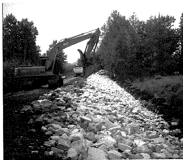
Placing riprap on enhanced river side slope
