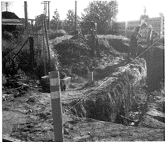
Excavation for tie-in to existing dyke
