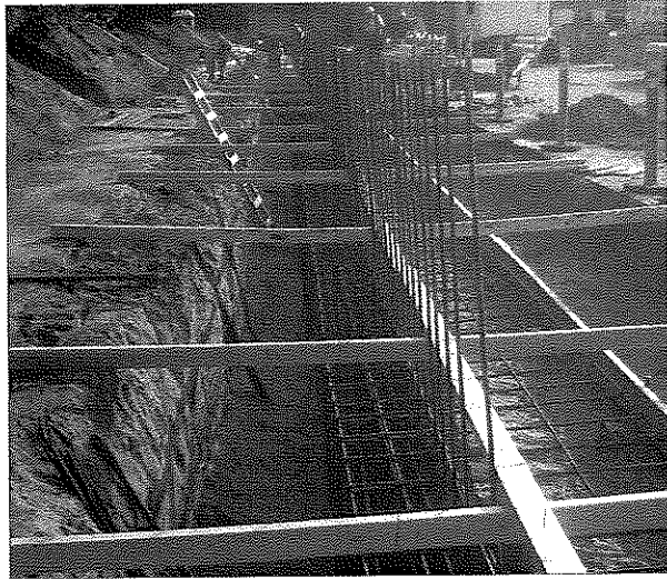
Forming and reinforcement
