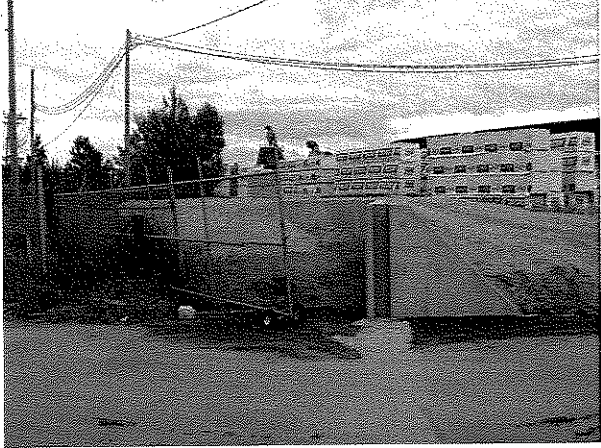
Finished concrete abutment wall
