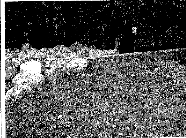
Tie in to adjacent high ground
