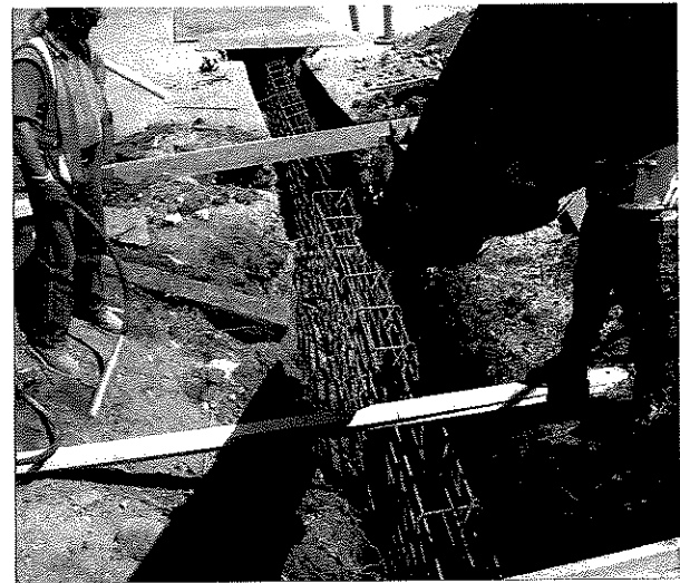
Reinforcing for buried seepage cut-off wall
