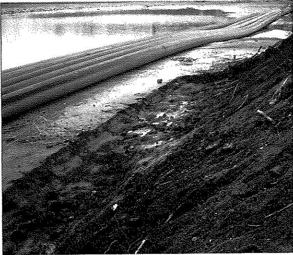
Stripping existing slope
