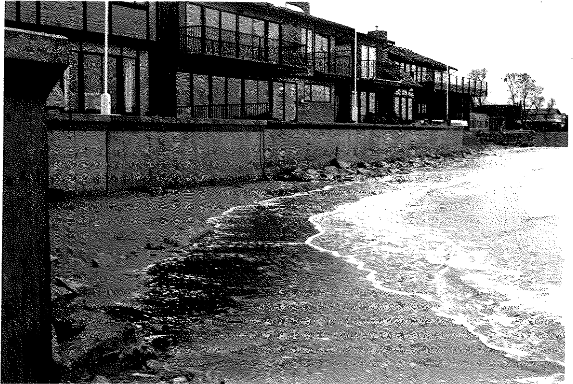
- Looking north from Canada - USA border - note riprap at toe of wall. 1984 12 13
