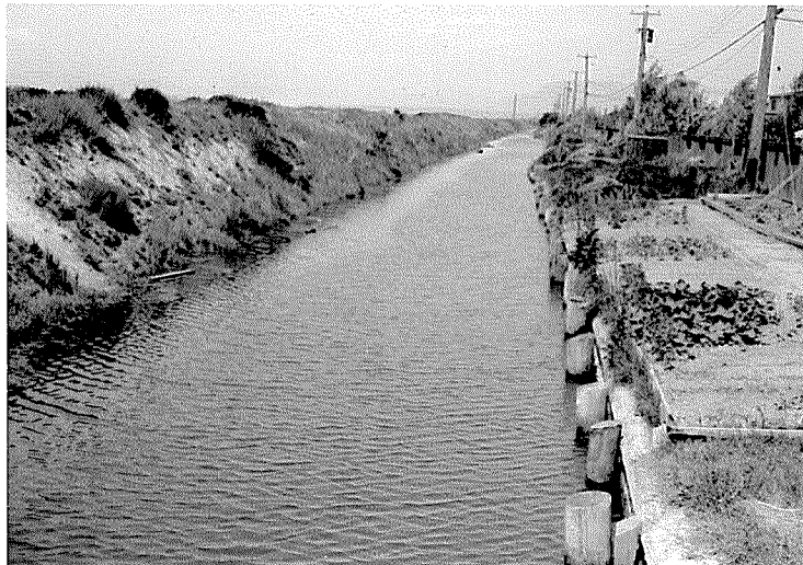
DITCH AND LANDSIDE OF DYKE LOOKING NORTH
