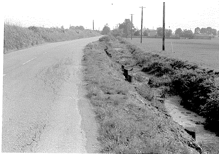
LULU ISLAND - MIDDLE ARM RIVER ROAD AT SECTION 1001
