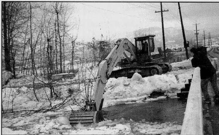
Ice Jam removal at bridge
