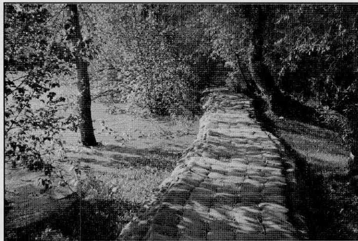
Sandbag dike at Mission Creek
