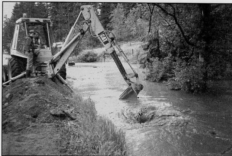
Clearing Culvert inlet at Coldstream Creek
