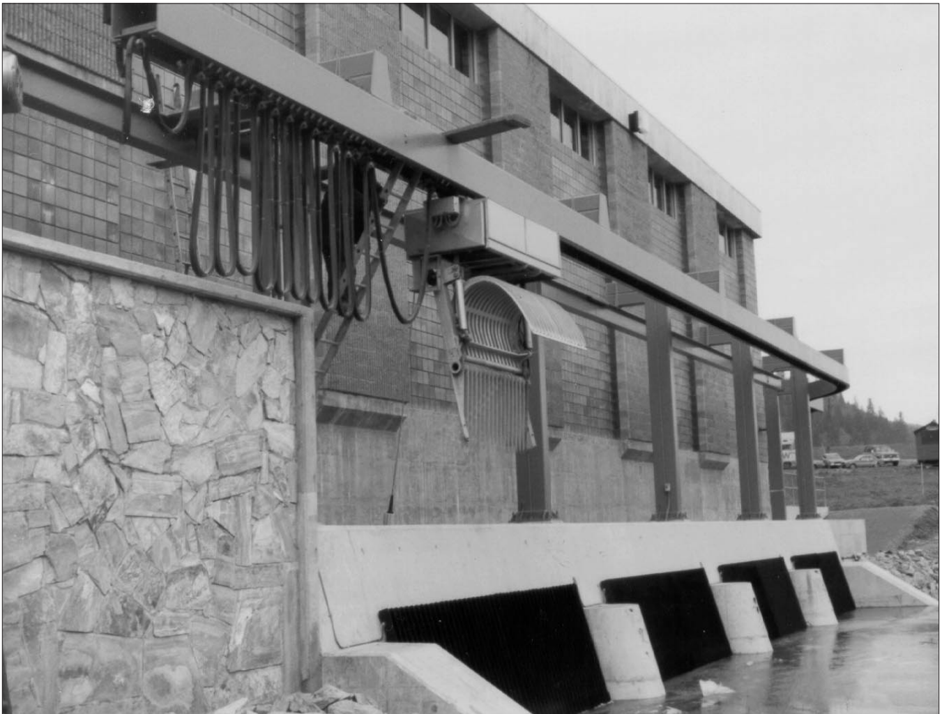
Barrowtown Pump Station
