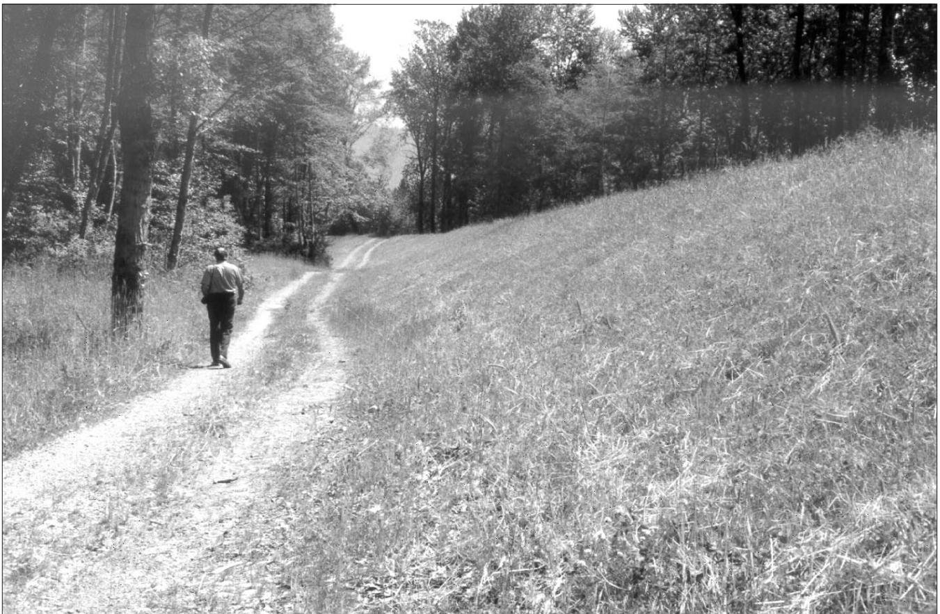
Inspecting the Landside Toe
