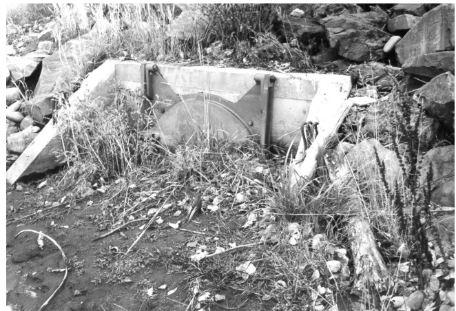
Blocked floodbox outlet.
