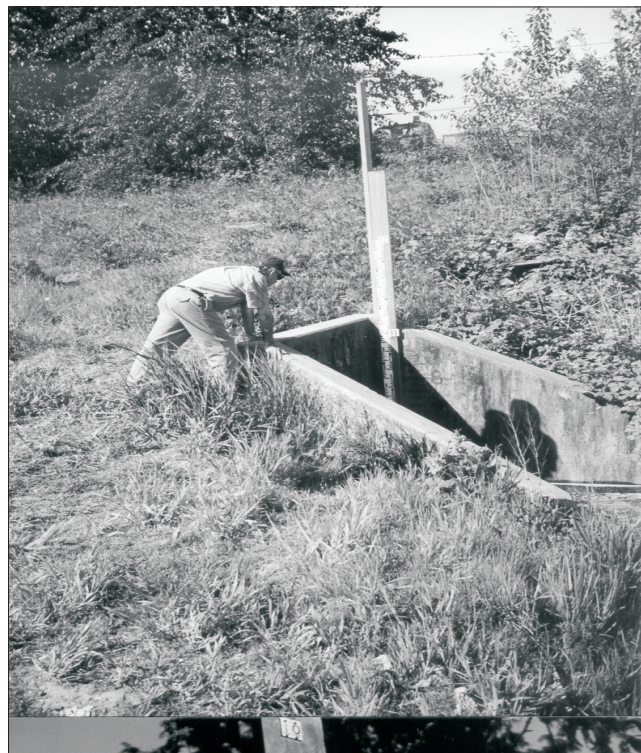
Inspecting a Floodbox
