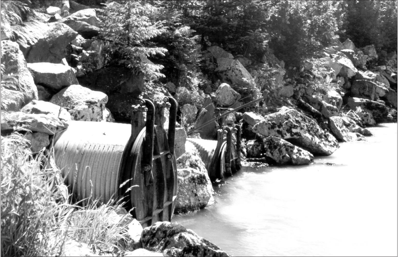
Uncontrolled Vegetation Growth on Erosion Protection Works.
