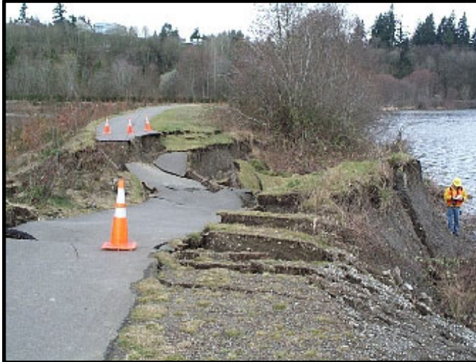
Dike Embankment Failure at Capitol Lake Nisqually Earthquake, February 2001
