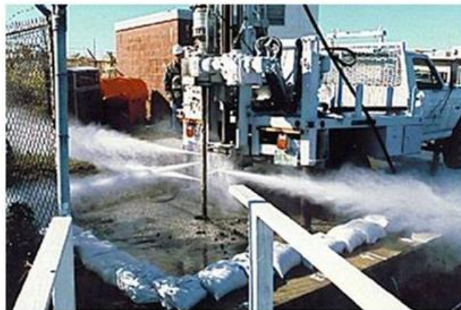
Figure C-4: Typical Jet Grouting Rig
