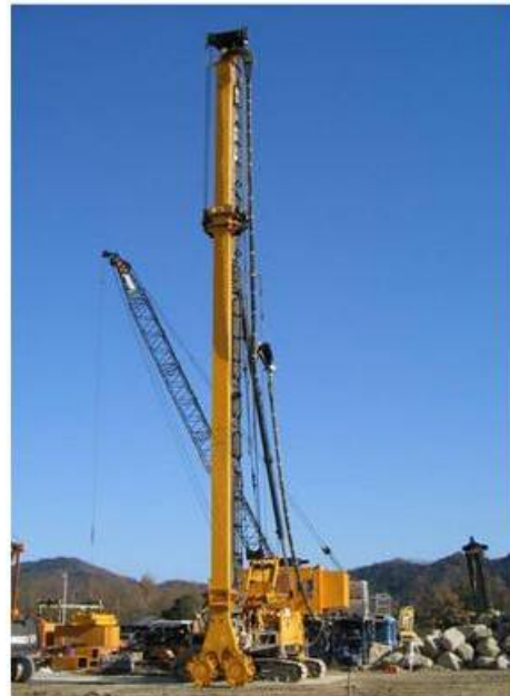
Figure C-6: Typical Soil Cutter Mix Rig
