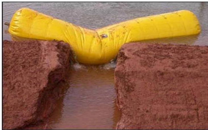
Figure D-1: Sample deployment of deep-breach closure system, with a small residual flow still persisting along the upper edges of the breach opening (Resio et al, 2008).
