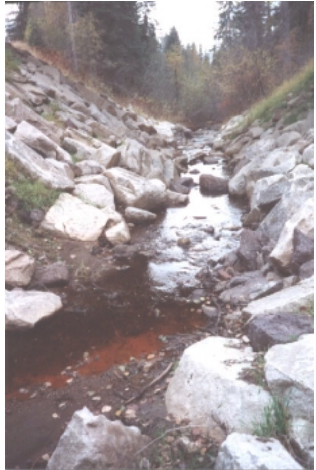
Photograph 5.01: Site 24, stream channel under the bridge, viewed from above the bridge. Note the highly constrained channel and steep rip rap armouring.
