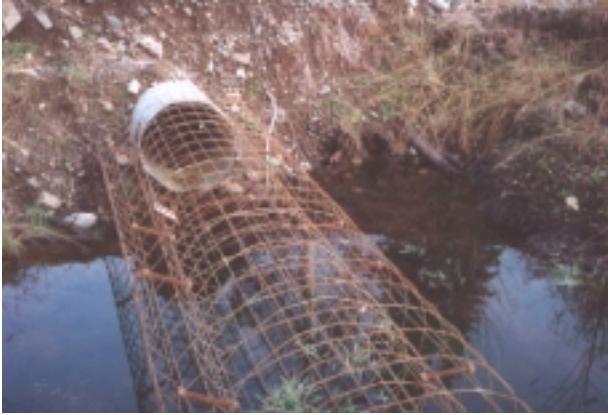
Photograph 10.02: Site 52, inlet. All the water is flowing through a crushed pipe to the right of the new culvert.
