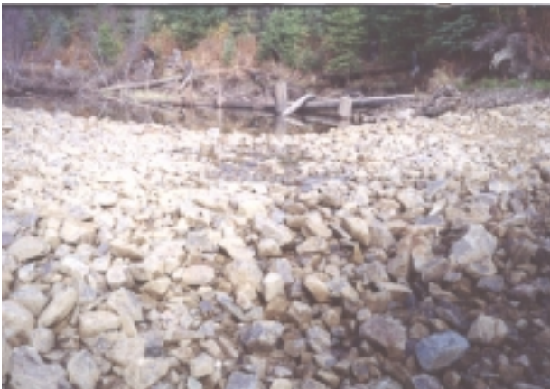
Photograph 7.10: Site 37, upstream view of ford showing rocks blocking fish passage.
