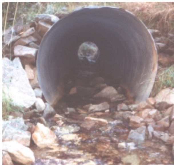
Photograph 6.04: Site 29, the culvert outlet in 2000, two years after remedial substrate placement.
