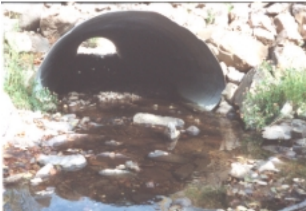
Photograph 2.07: Site 9, culvert outlet. Note ponding at the outlet resulting from high outlet water velocity.
