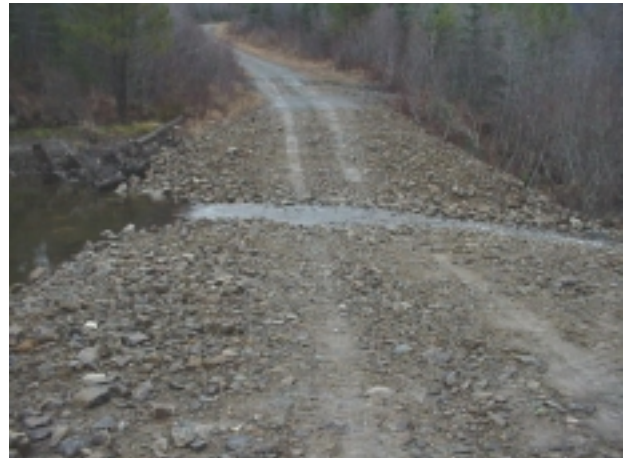
Photograph 0.02: Site 37, ford modified to permit fish passage (current speed at peak flows may be an issue). Pickup access to the ford has been blocked to prevent sedimentation..
