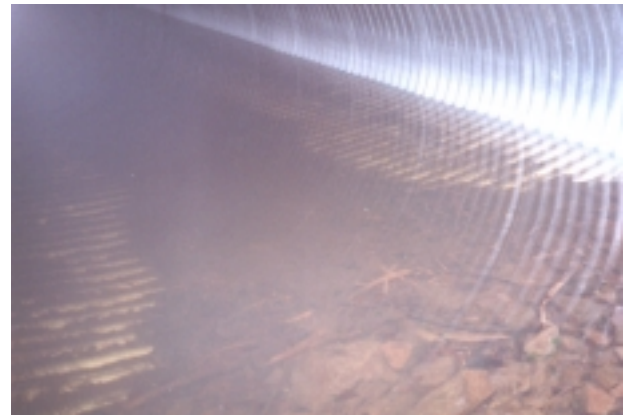
Photograph 11.11: Site 60, interior of culvert. Note that much of the substrate has flushed out of the pipe.
