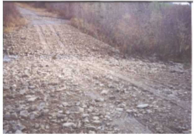
Photograph 7.12: Site 37, ford blocking fish passage from use of uncompacted rock.
