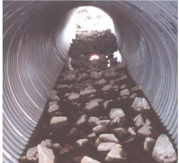
Photograph 4.07: Site 19, interior from outlet. Note the rock near the inlet is blocking fish passage.
