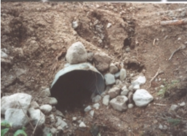
Photograph 2.10: Site 11, culvert inlet. Note the erosion of the road surface and roadbed.
