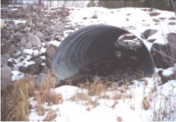
Photograph 15.07: Site 7, outlet. Note that little substrate remains within the culvert.
