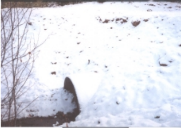
Photograph 11.13 (above): Site 61, culvert outlet with roadbed failure.
