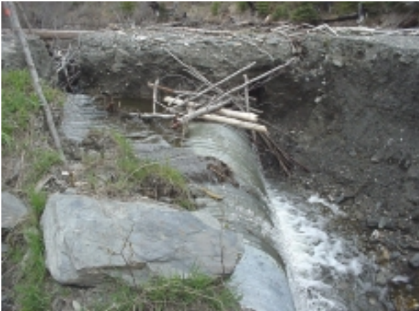
Photograph 0.01: Site 37, washed out culvert (beaver plugged).
