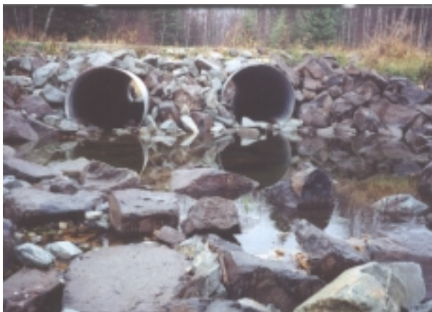
Photograph 8.07: Site 43, retrofitted culvert crossing. Culvert width = 1.6 m ; 1.8 m; Culvert slope = 1%.
