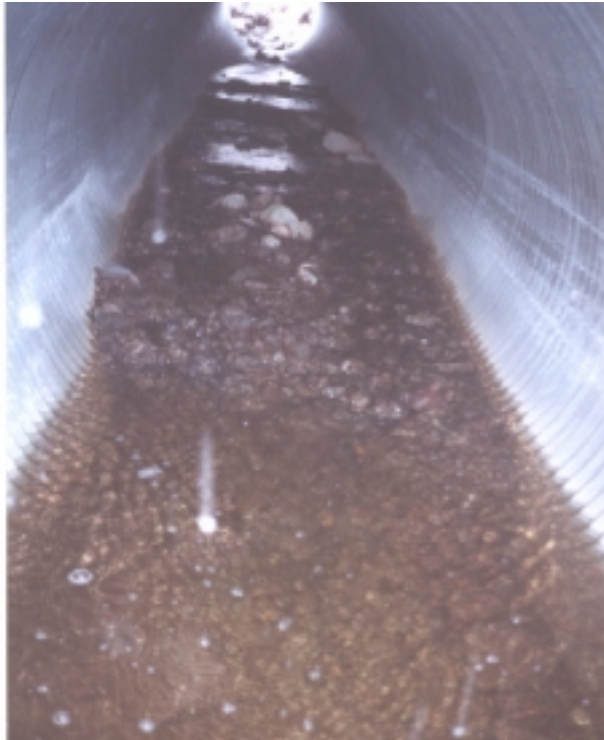
Photograph 10.04: Site 54, interior from outlet. Note that much of the substrate has flushed from the outlet end.
