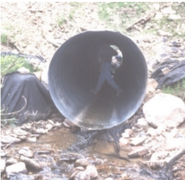
Photograph 0.05: Site 29, original 1998 installation showing perched outlet and lack of substrate in the pipe.
