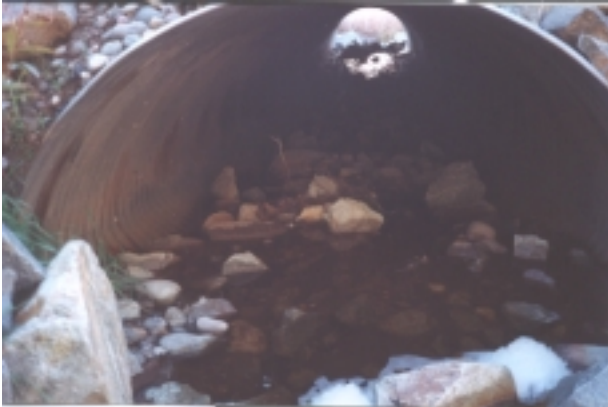
Photograph 5.13: Site 28, outlet. Note that some of the substrate has flushed out despite large rock size. Stream width = 0.5 m Culvert width = 1.5 m Culvert slope = 3%
