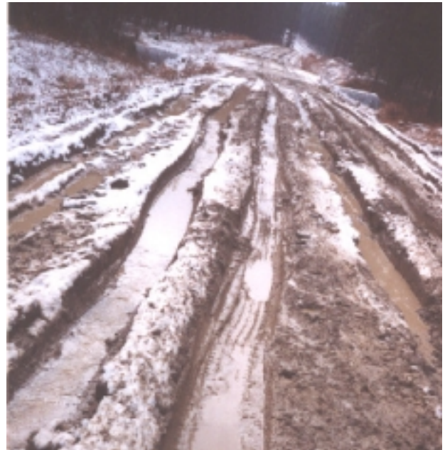
Photograph 11.05: Site 59, sediment from road surface is entering stream (the culvert in right background).
