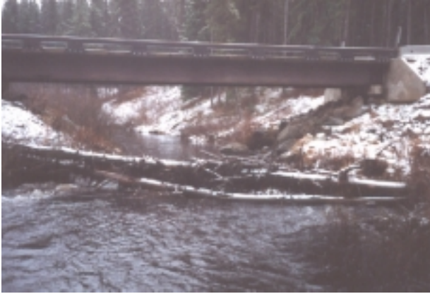
Photograph 10.12: Site 57, bridge. The logjam is downstream of the bridge, and hence is not of concern.
