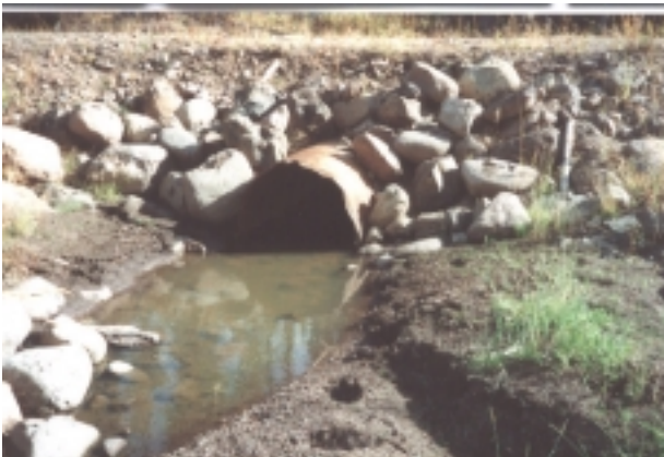
Photograph 2.08: Site 10, culvert outlet. Note the ponding at the outlet that has resulted from scouring.
