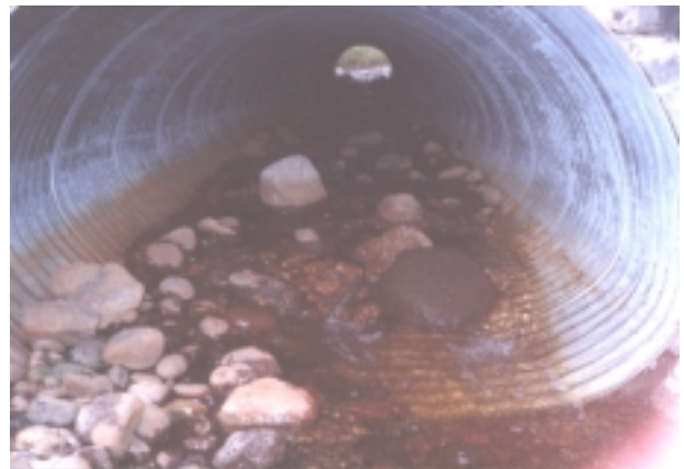
Photograph 4.03: Site 18, interior from outlet. Note that the substrate has flushed out of part of the lower end of the culvert; some scouring has occurred below the pipe. Stream width = 1.2 m Culvert width = 1.5 m Culvert slope = 5%
