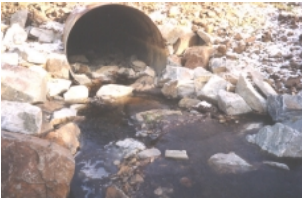
Photograph 5.11: Site 27, inlet of culvert, fish passage blocked at low water by rock substrate.
