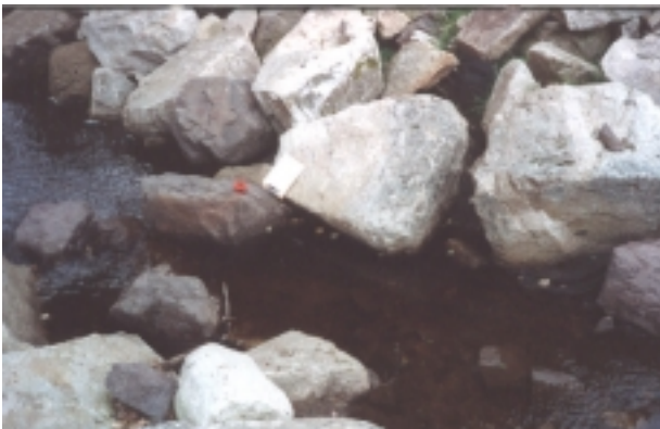
Photograph 5.02, Site 24, rip rap slipped into channel. Note white clipboard for scale.
