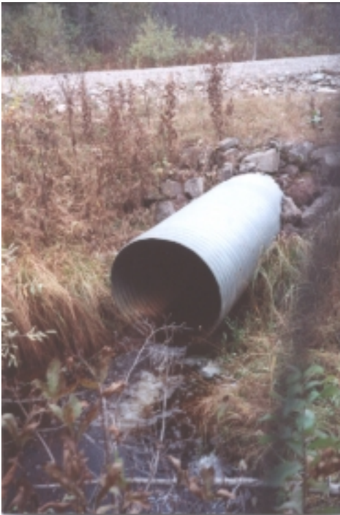
Photograph 5.06: Site 25, outlet showing plunge.
