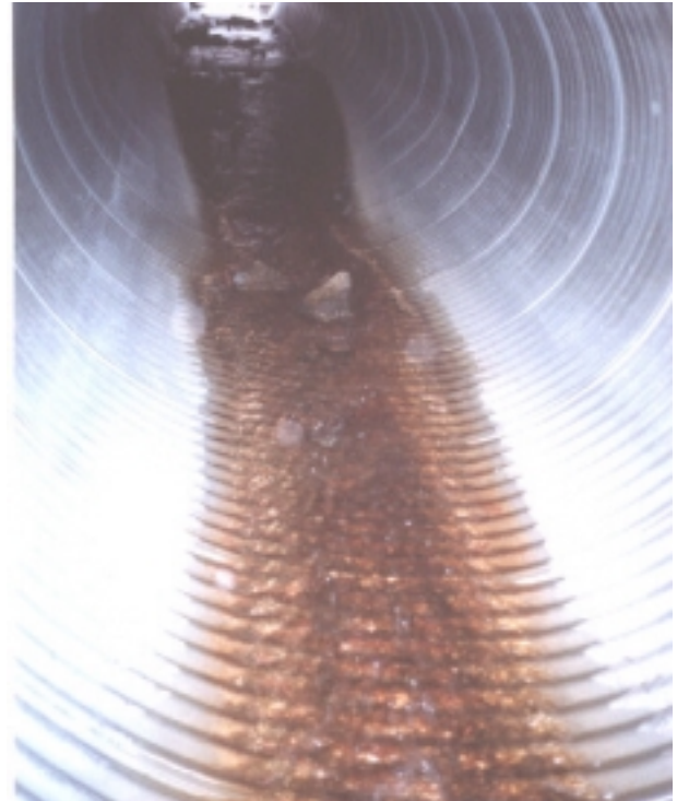
Photograph 10.05: Site 54, interior from inlet. Note the substrate has flushed out of the top end of the pipe.
