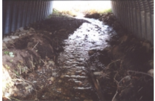
Photograph 8.19: Site 47, interior from inlet. The full width of the arch near the outlet is floodplain.
