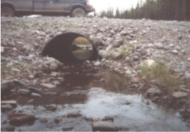
Photograph 3.: Site 14, outlet. Stream width = 2.0 m Culvert width = 2.0 m Culvert slope = 0%
