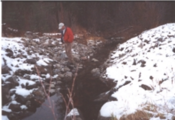
Photograph 12.10: Site 4, armoured ford for ATVs.
