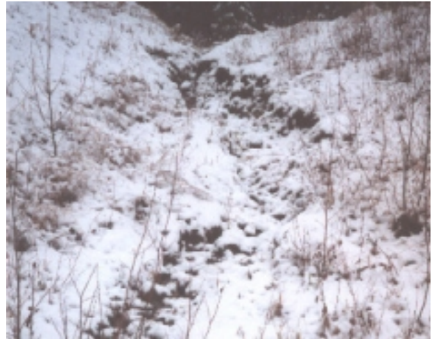
Photograph 10.09: Site 55, ditchline eroding into stream (stream just below bottom edge of photograph).
