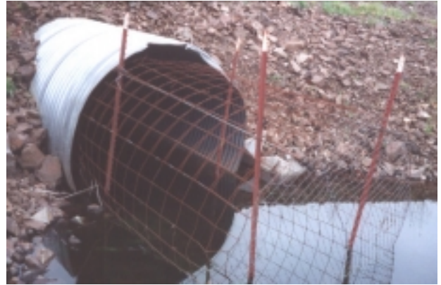
Photograph 0.01: Site 26, inlet with "beaver stop".
