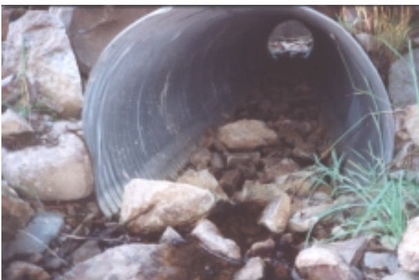
Photograph 6.09: Site 30, inlet. Note that large rocks used as substrate impede fish passage.
