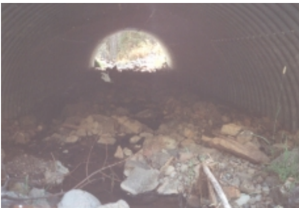
Photograph 2.02: Site 8, interior from inlet, showing eroded substrate.
