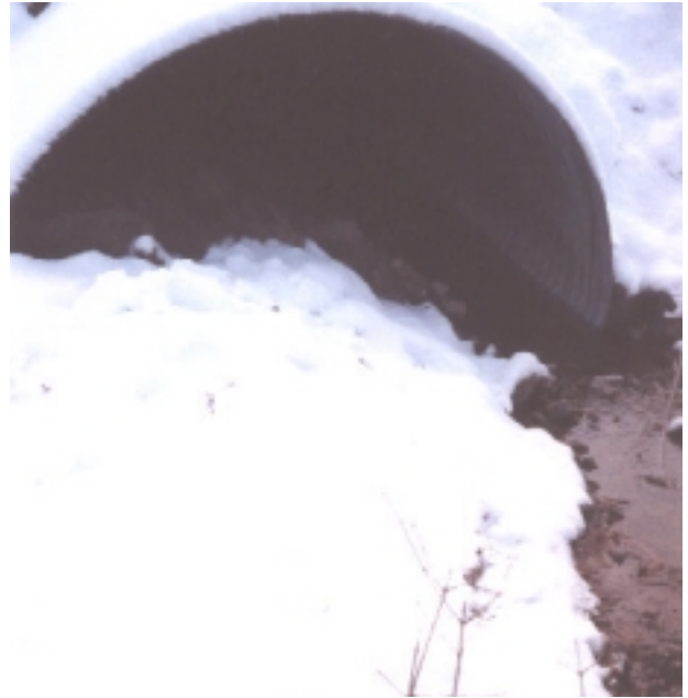
Photograph 11.12 (to right): Site 61, culvert outlet partly filled with roadbed material.
