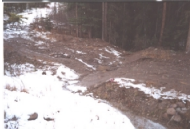
Photograph 12.12: Site 4, cross-ditch above the stream. Sediment will be delivered directly into the stream.
