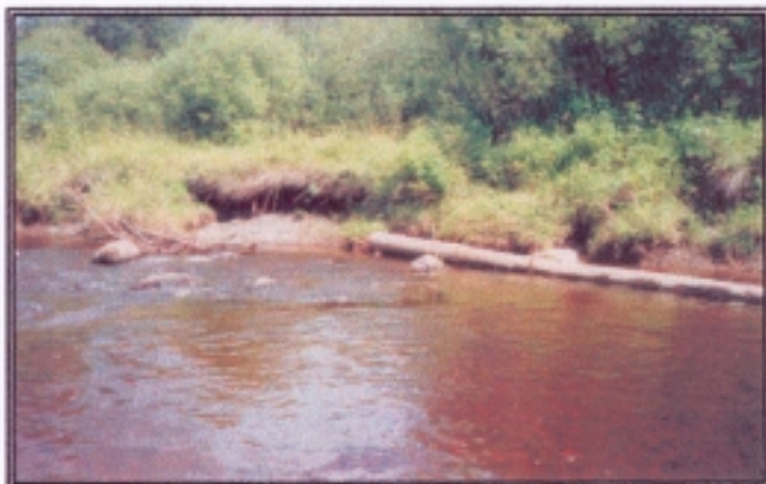
Downstream view. Note scour at downstream end of structure.
