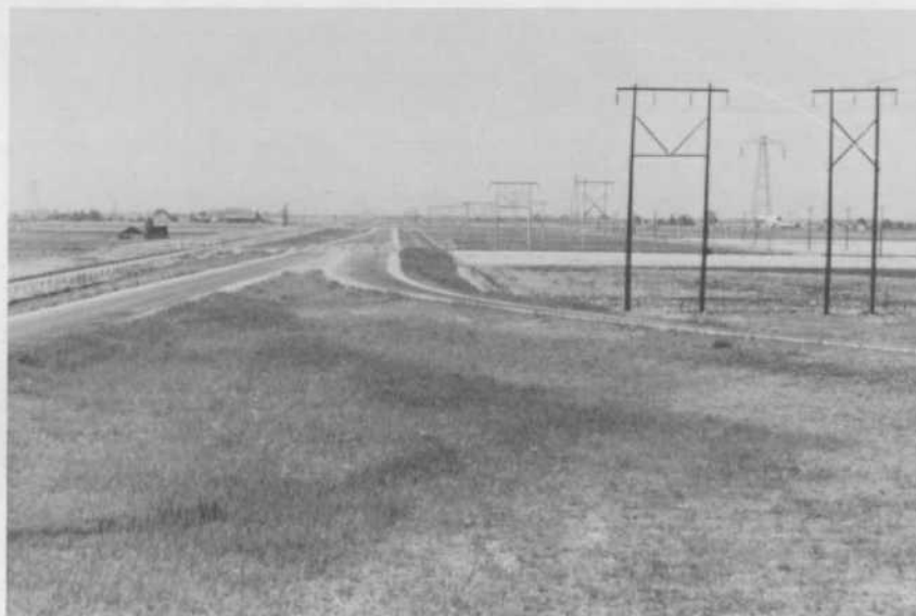
Plate 47 Transportation and utility corridors occupy substantial lands in the Langley-Vancouver map area. This view in Delta Municipality is an example.
