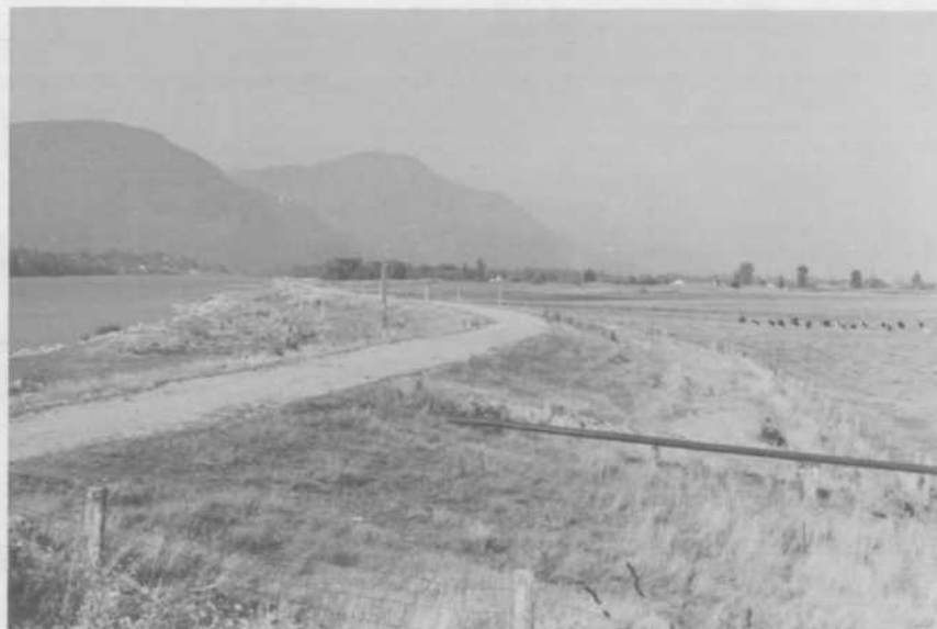
Plate 3 Dyke along the Fraser River in Matsqui valley. The lowlands of the Lower Fraser Valley are protected from periodic flooding by an extensive system of dykes.
