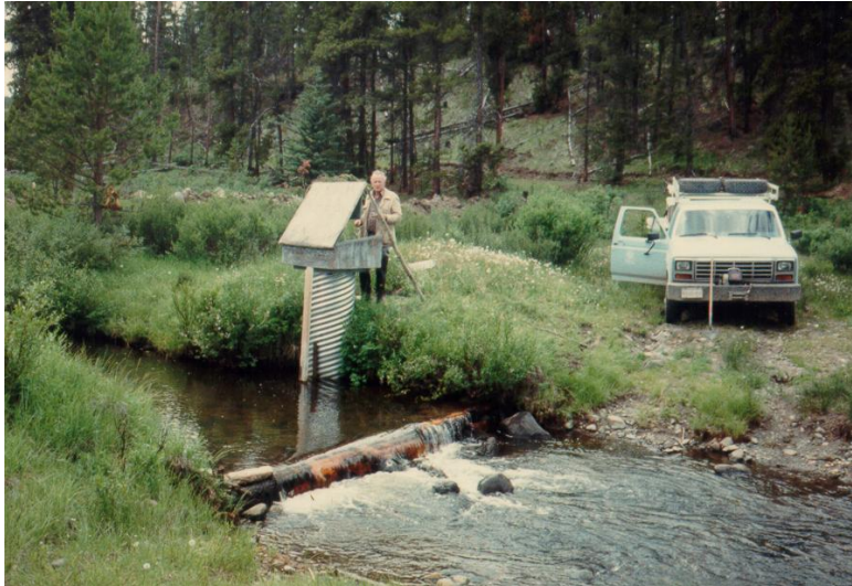
Figure 5: A Stable artificial control (log sill).
