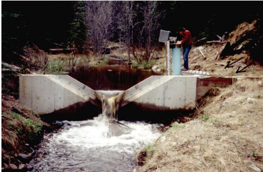
Figure 65: Stilling well installed in the weir pond.
