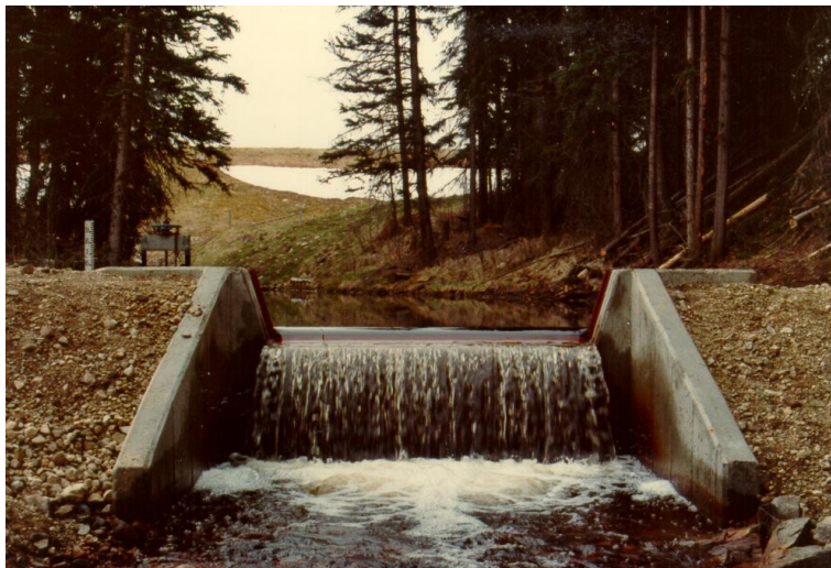
Figure 4: A Stable artificial control (weir).
