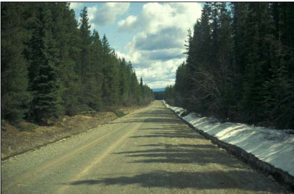
Forest service road, Ft. St. James District. Photo: Phil Burton
