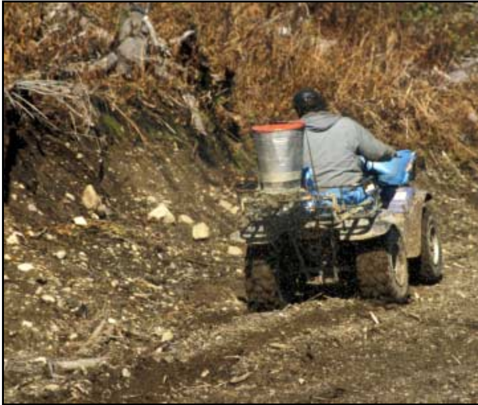
Figure 12. Dry broadcast seeding along a newly built logging road, spreading a grass-legume seed mix using a cyclone seeder mounted on an all-terrain vehicle (ATV).
