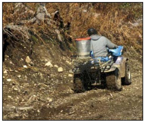
**Figure 12.** Dry broadcast seeding along a newly built logging road, spreading a grass-legume seed mix using a cyclone seeder mounted on an all-terrain vehicle (ATV).
