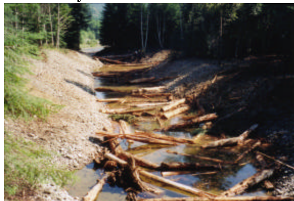
Figure 1. Constructed LWD cover structure in Tributary G02.
