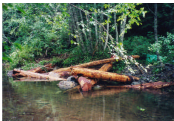
Figure 1. Constructed LWD cover structure in Tributary G02.
