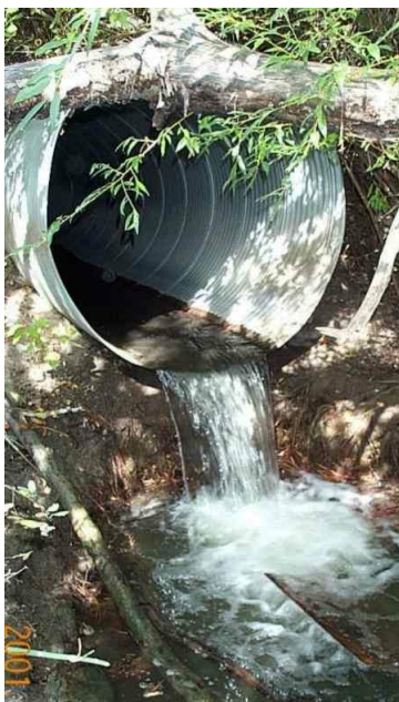
This perched culvert is a barrier to fish passage T. CASHIN PHOTO
