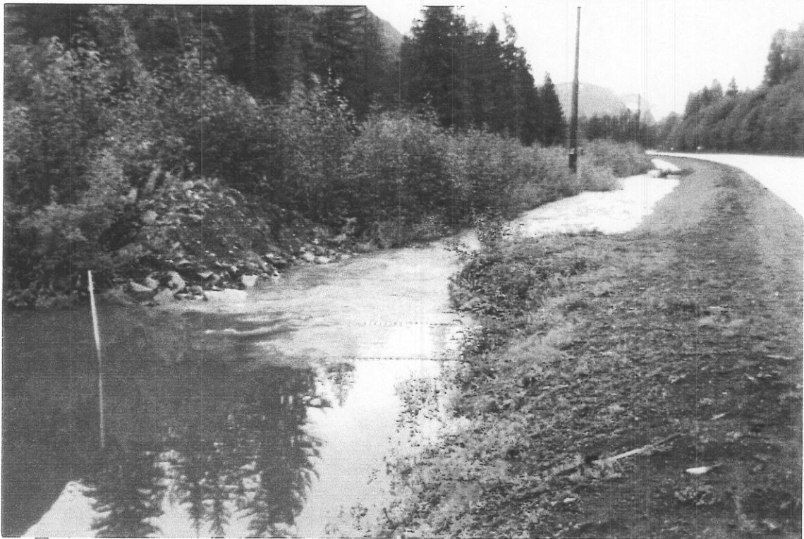
PHOTO 20: FLOW REVERSAL AT CULVERT CROSSING OF HIGHWAY 37A, 70 M DOWNSTREAM OF CROSS SECTION 29 HAY & COMPANY CONSULTANTS INC.
