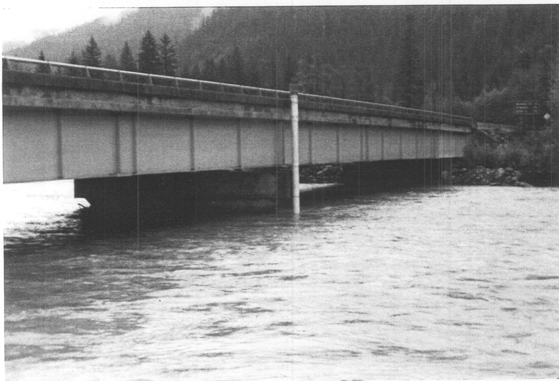
PHOTO 15: BEAR RIVER BRIDGE WITH WATER MANAGEMENT DIVISION GAUGE ON DOWNSTREAM FACE
