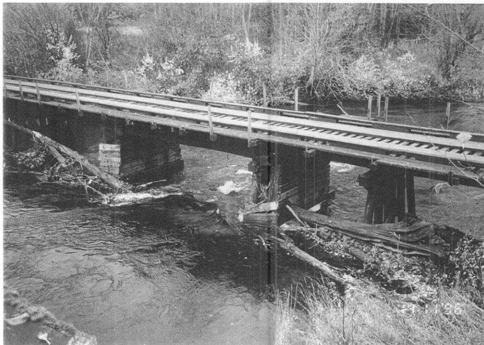
Photo 41 Looking downstream from abandoned M&B haul bridge to XS-27 along upstream edge of former rail bridge. Note debris buildup.
