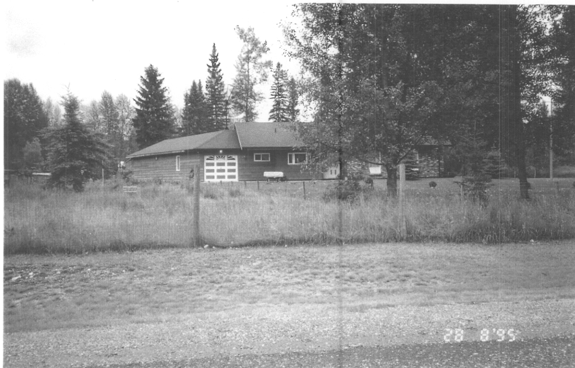
Photo 9: Naver Creek - Recently constructed home vicinity of XS 7 & 8 Note use of fill to achieve some flood protection
