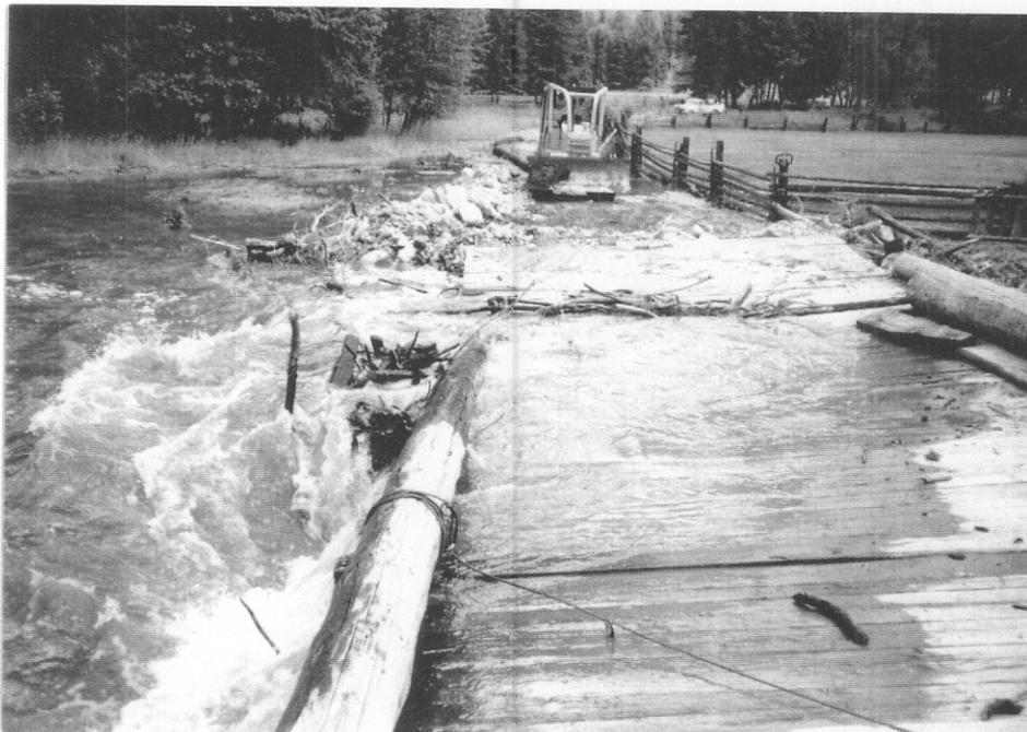
Photo 2 Attempts to save a driveway bridge during the June 1990 flood. Looking toward the left abutment along the upstream side of the bridge at cross section XS-260.
