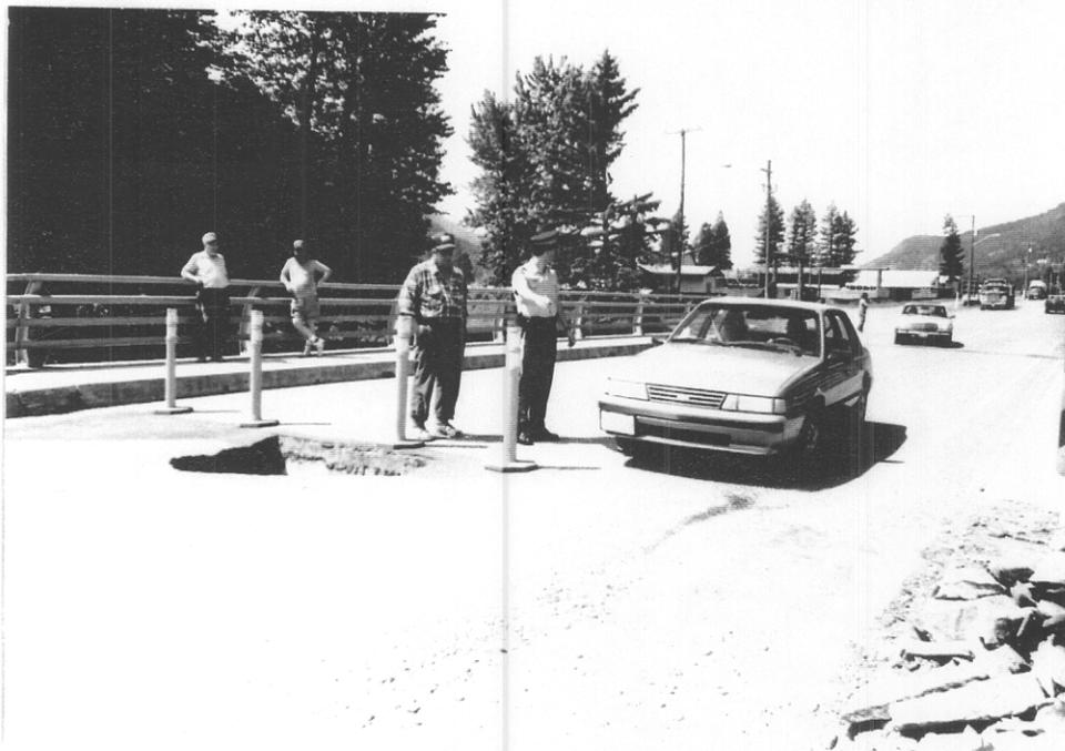
Photo 7 A hole in the pavement at the left abutment of the Highway 97 bridge over Bolean Creek caused by undermining by flood flows, June 1990.
