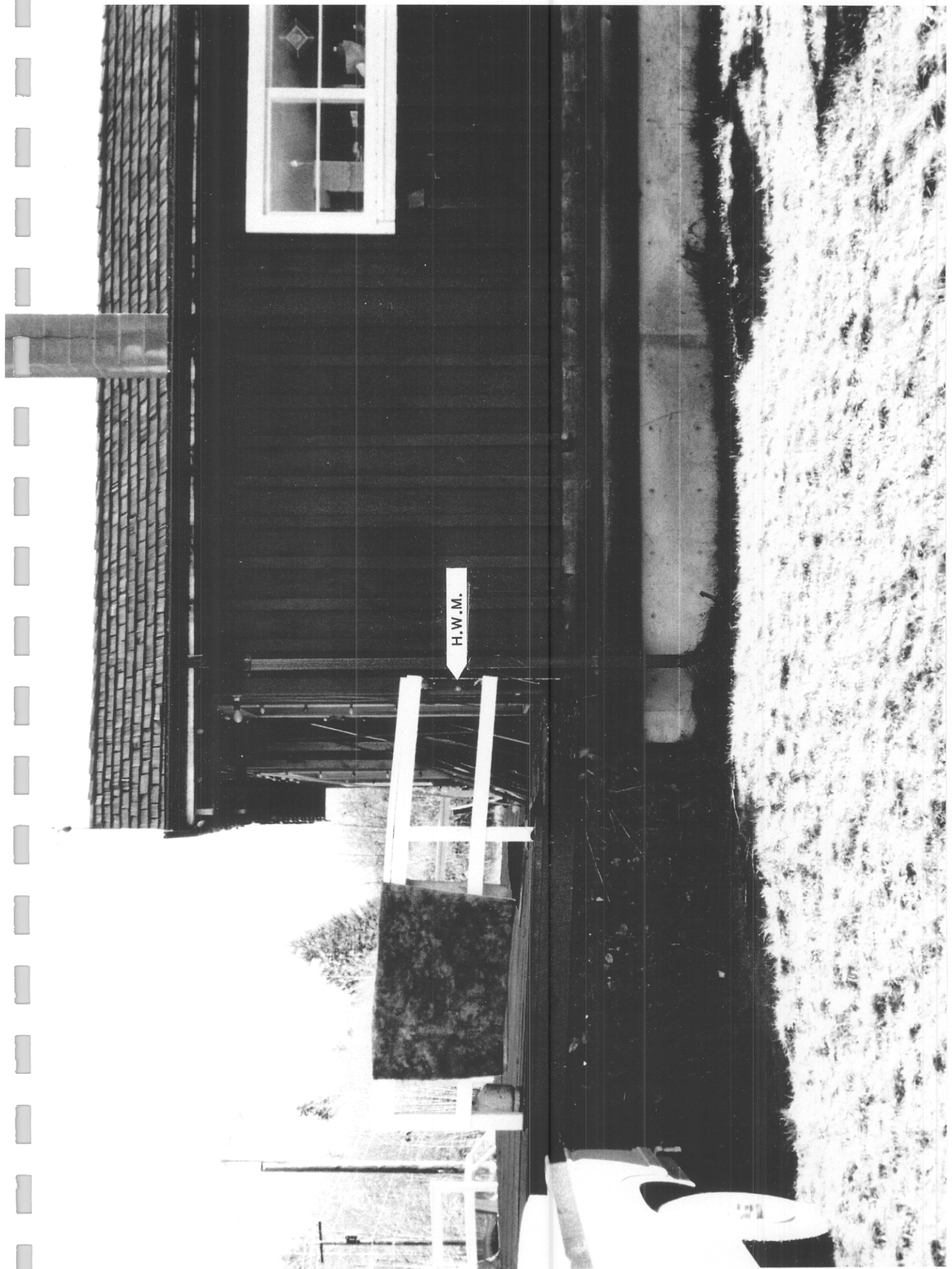
PHOTO 1: SALMON RIVER AT SAYWARD - HOME FLOODED NOVEMBER 11 AND 23, 1990 NOTE H.W.M. BETWEEN DECK RAILS
