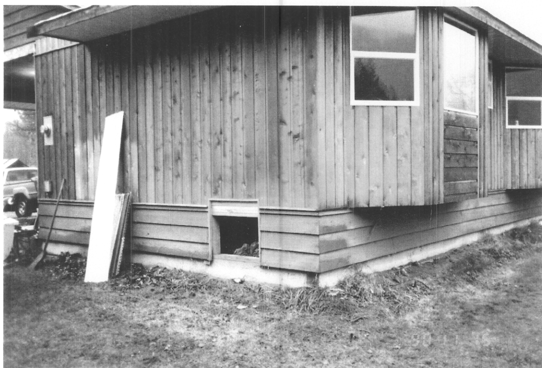
PHOTO 3: HWM 90-29 - TOP OF FRAME AROUND ACCESS DOOR - HOME LOCATED AT THE FOOT OF ARMISHAW ROAD (NOTE THIS HOME WAS FLOODED DURING THE 1975 EVENT AND SUBSEQUENTLY RAISED ABOUT 2 FEET)
