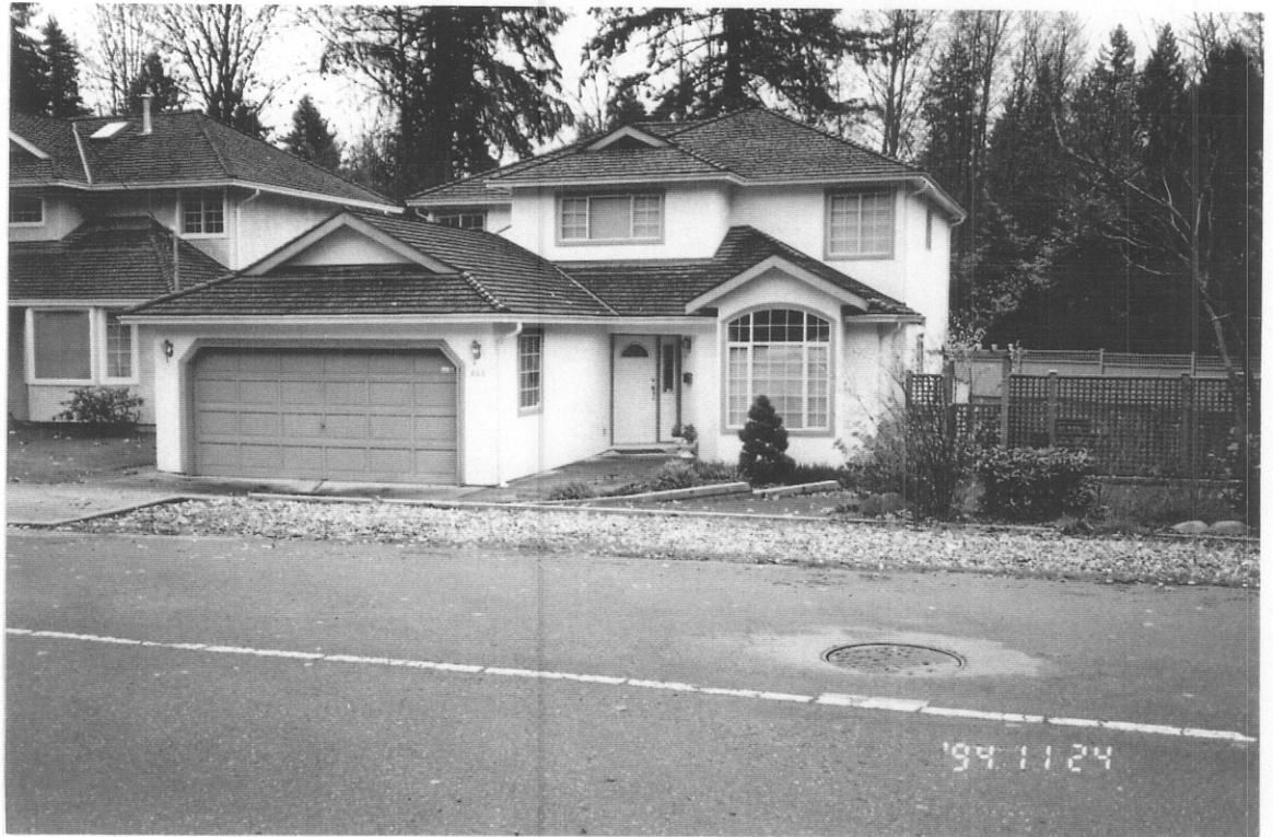
17. Looking southeast at 660 Seymour Boulevard, which is west of the house in photo 16. This house appears to be constructed at the natural ground elevation below road level and is approximately one metre lower than an older home (not shown) on the downstream side.
