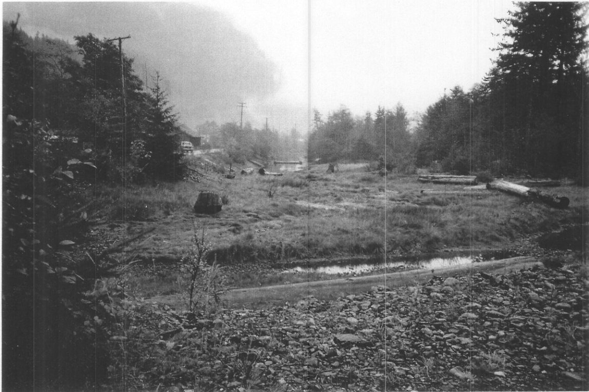
ZEBALLOS (Photo 10) Former Zeballos river channel blocked off with dyke in 1940/41. Channel partially infilled by Zeballos Iron Mines for access road to wharf (now called Pandora Crescent).
