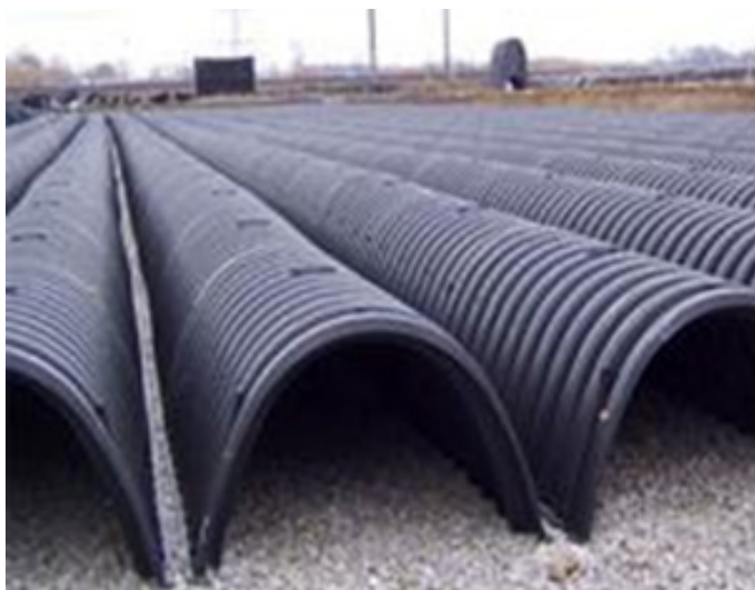
Figure 4: Example of proprietary underground percolation systems
