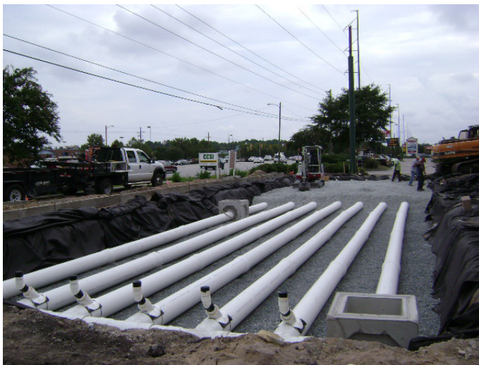
Figure 3: Infiltration trenches are non-proprietary underground percolation systems
