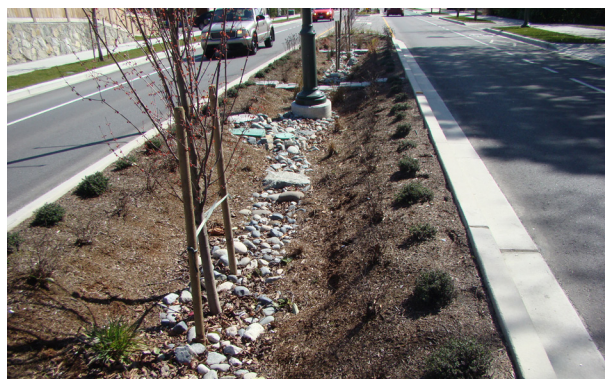
Figure 1: Bioretention areas (left) and swales (right) are common surface infiltration practices
