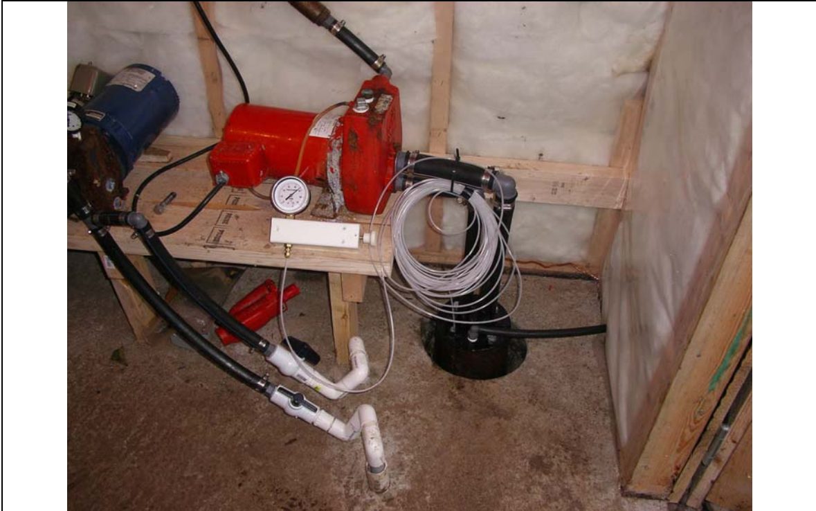
Photo 3. Well 1 with air-line installed.
